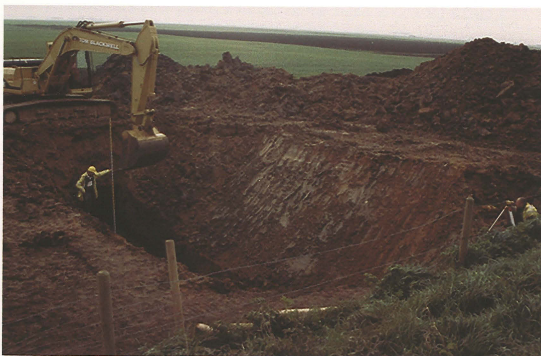
Plate 2: Construction of thrust pit to the north of Car Dyke
