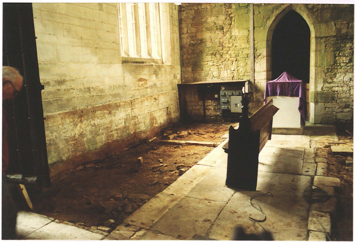
Pl. 11 Area 3 general view after removal of pew platform and before cleaning looking west
