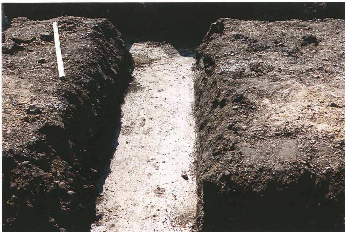
10.2.2 View of the main building foundations infilled with concrete
