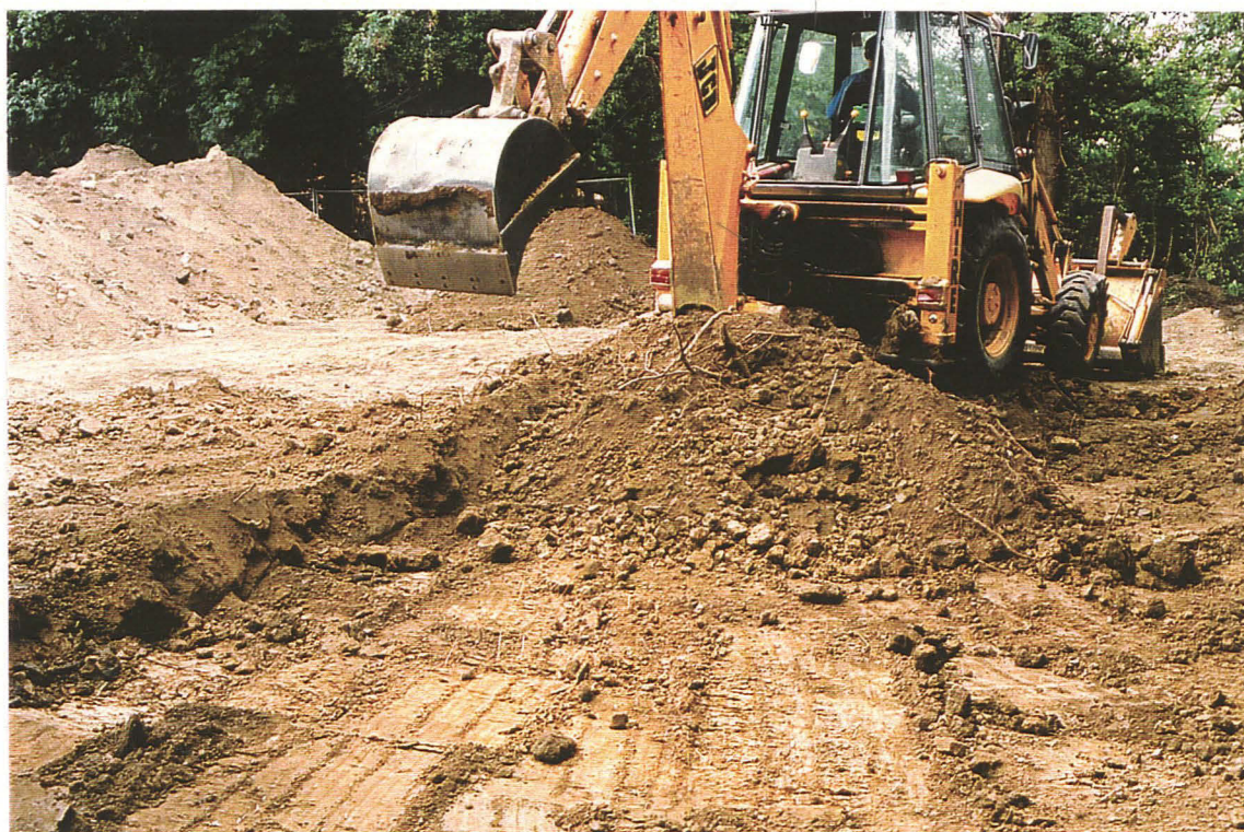
10.2.5 View of the soakaway being excavated with 'battered' edges, north-east facing.
