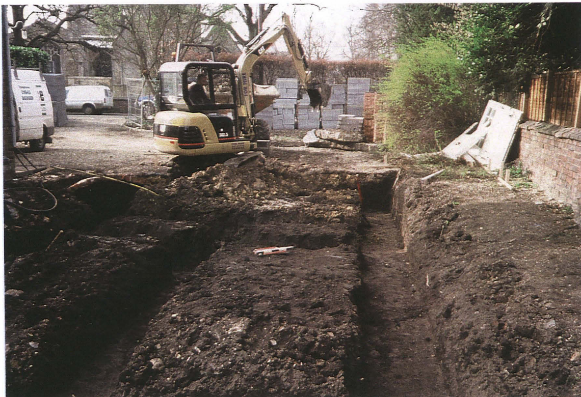
8.2.1 Extension footings, facing north west.
