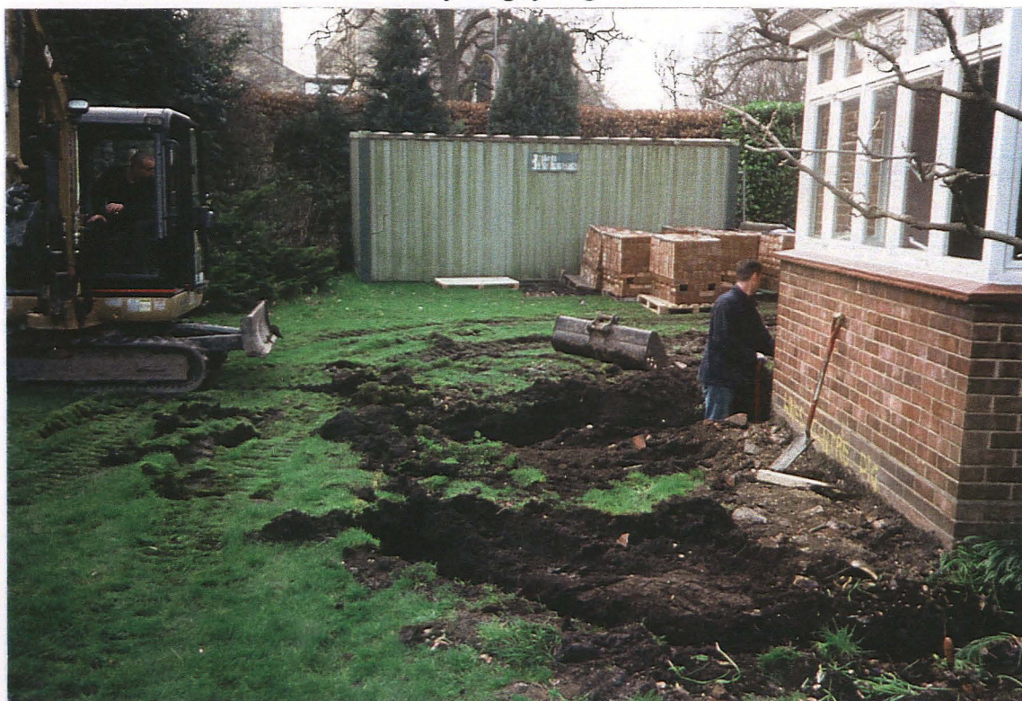
8.2.2 Conservatory footings, facing north west.
