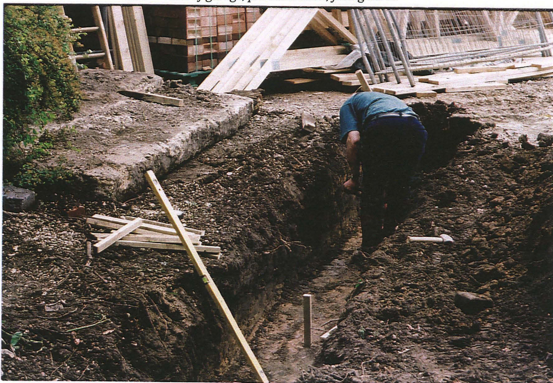
8.2.4 Garage footings, facing west.
