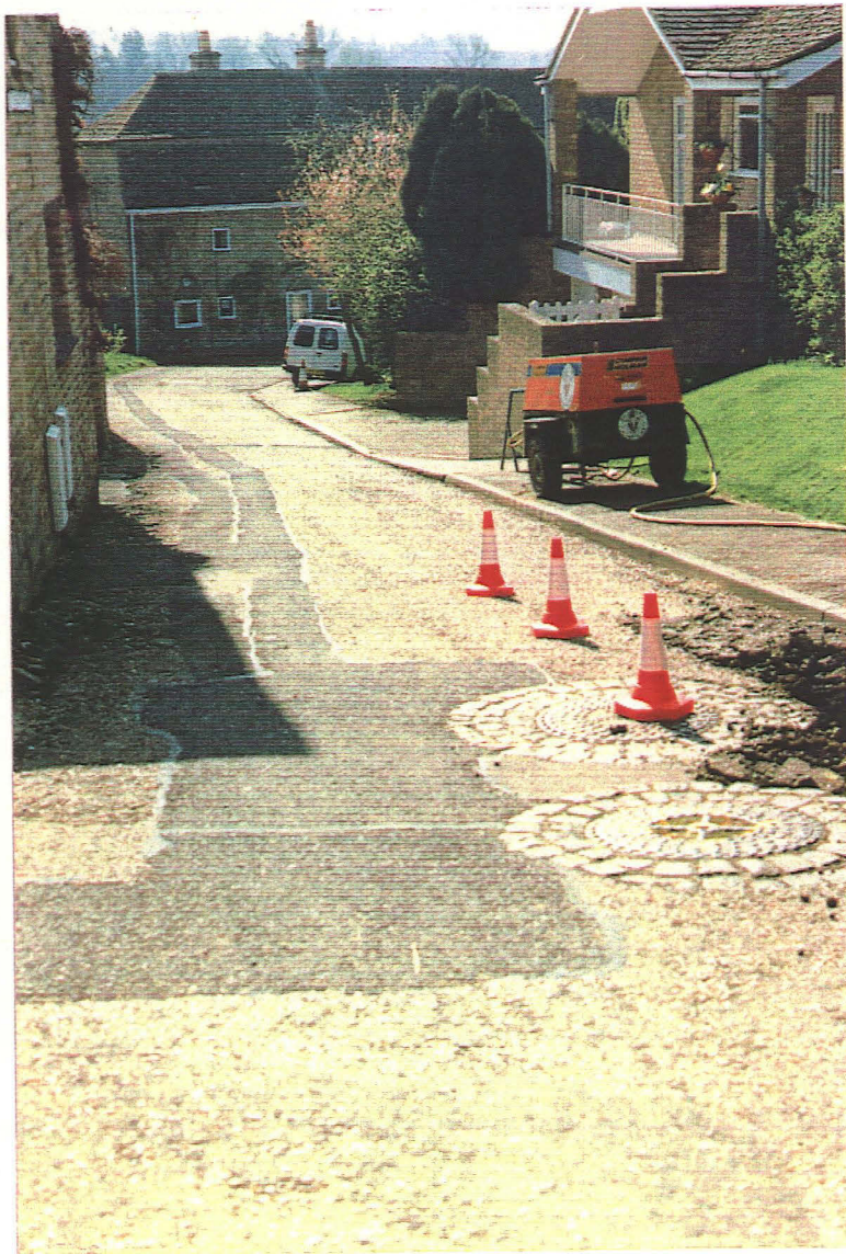
Plate 1. Austin Friars' Lane Before the Construction of the New Sewer Link.
