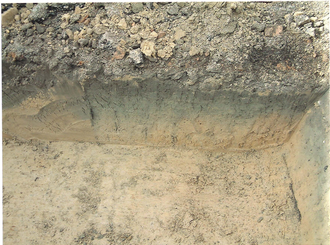
Plate 6. Section showing contamination in trench 2.
