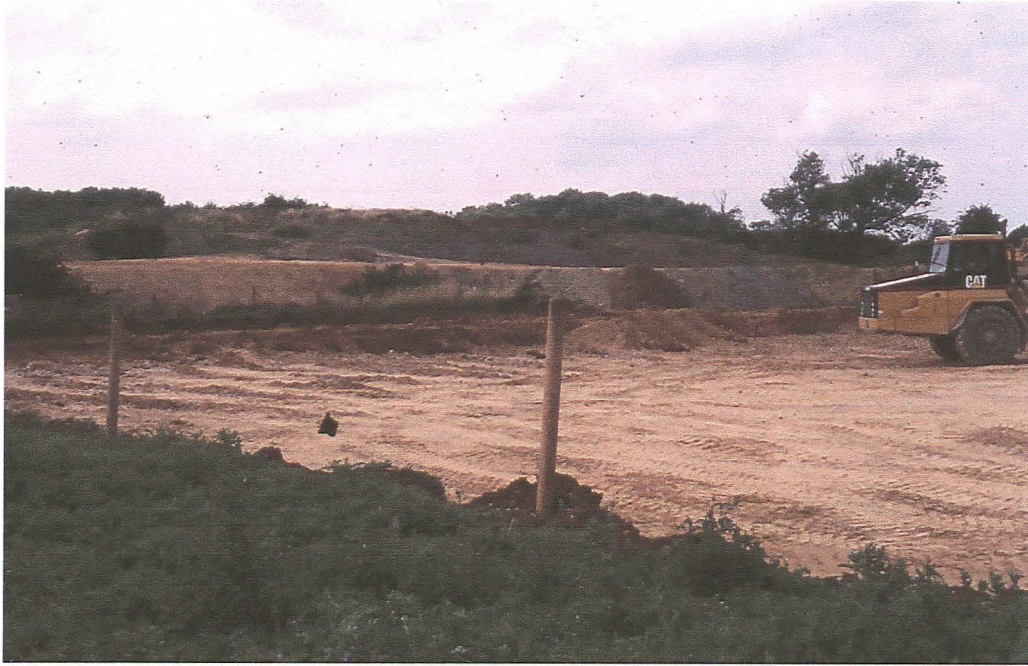
Plate 1: General view of work in progress
