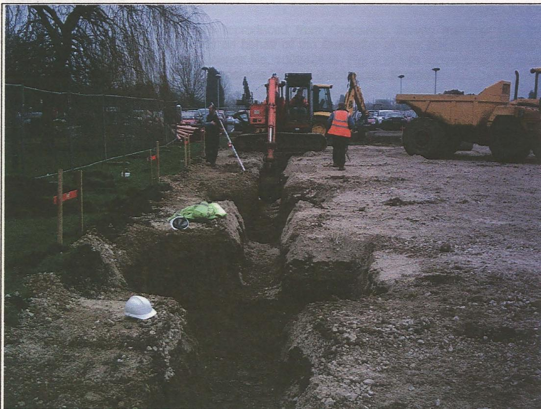
Plate 1: General view showing the excavation of groundbeams for the new sports hall (looking east).
