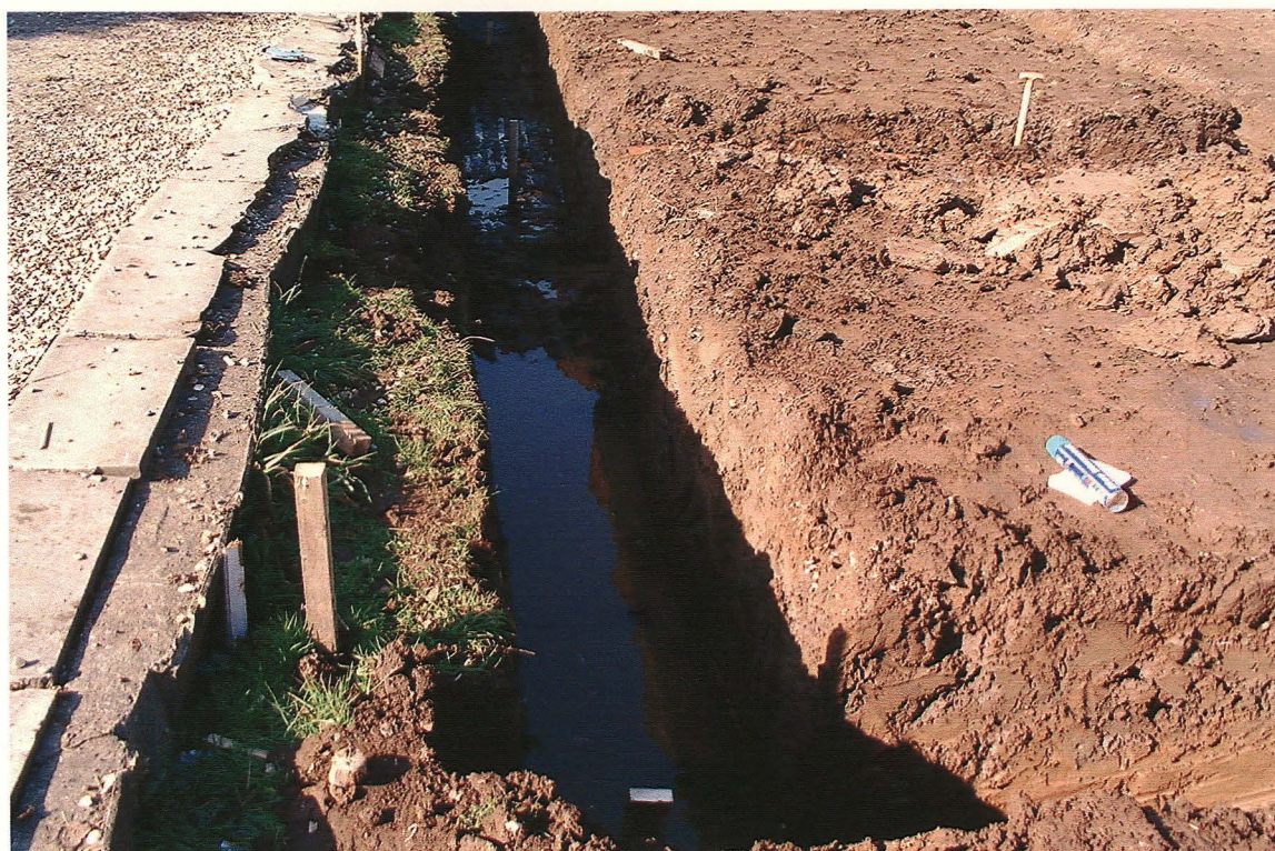
Plate 5. Showing increased depth of footings to south side of site and water table.
