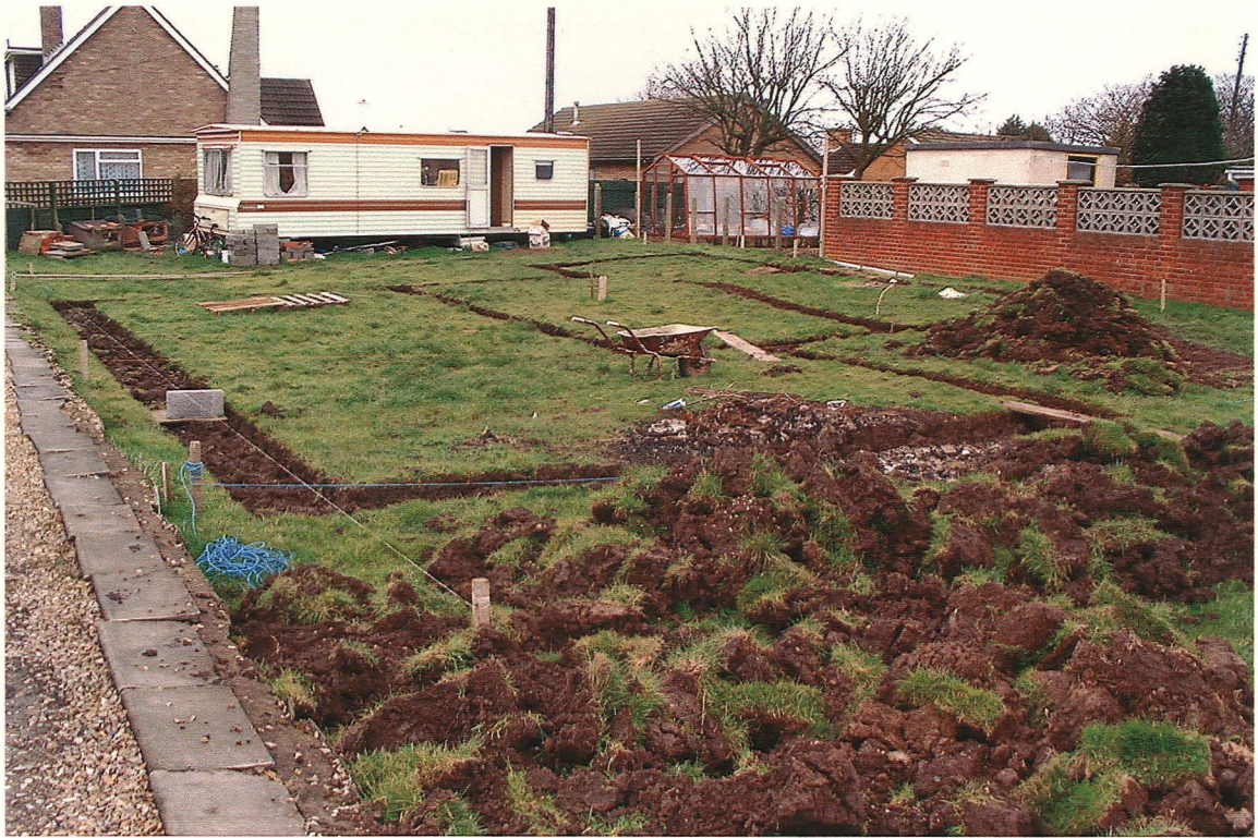
Plate 1. Site prior to excavation.
