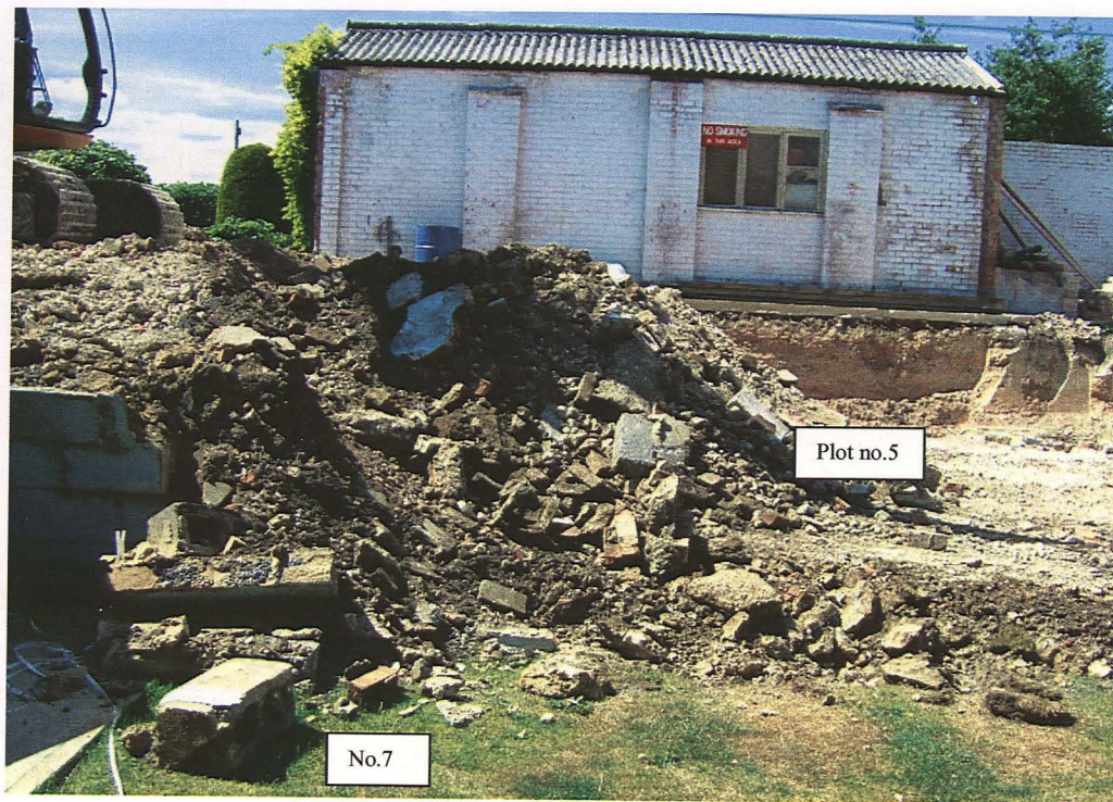
Plate 27: Boundary wall dividing plots nos.7 & 5 during demolition programme; looking west from plot no.7.
