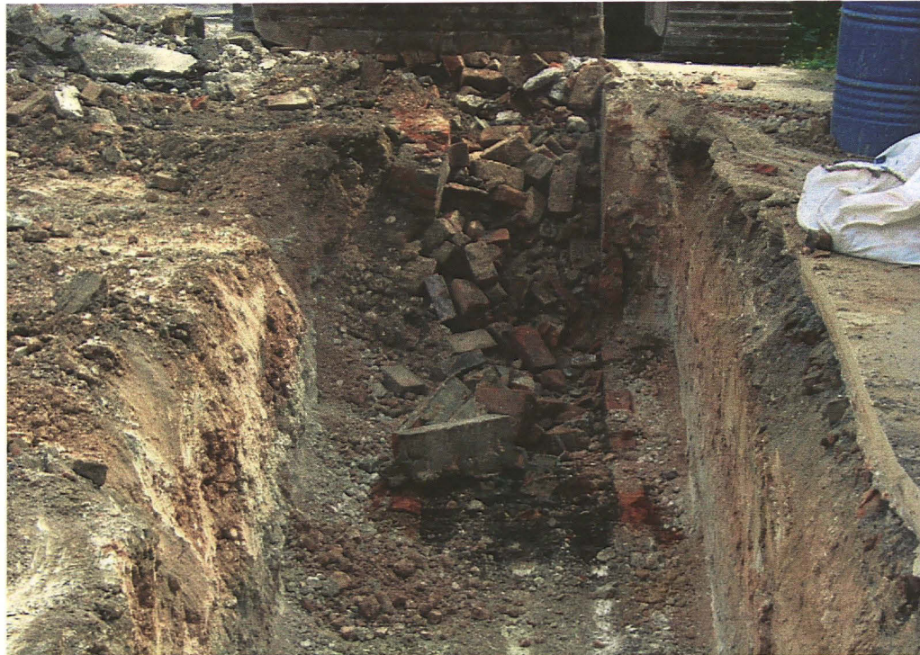
Plate 22: Excavation of brick-lined pit and removal of backfill; looking south.
