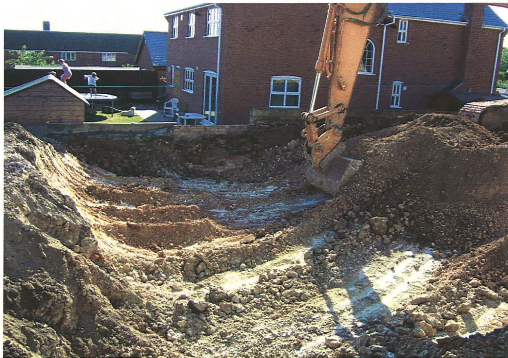
Plate 16: View across former warehouse structure following machine excavation showing the red clay subsoil and underlying chalk; looking east.
