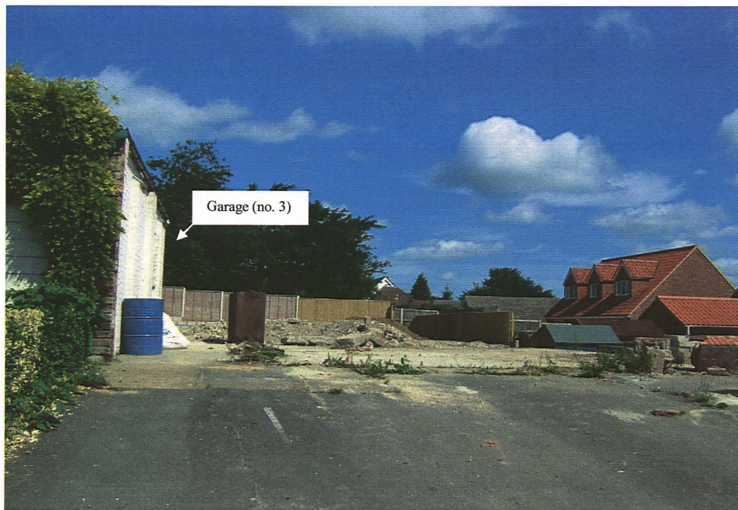
Plate 4: View of plot no.5 from South Rise road looking north, prior to the start of ground works.
