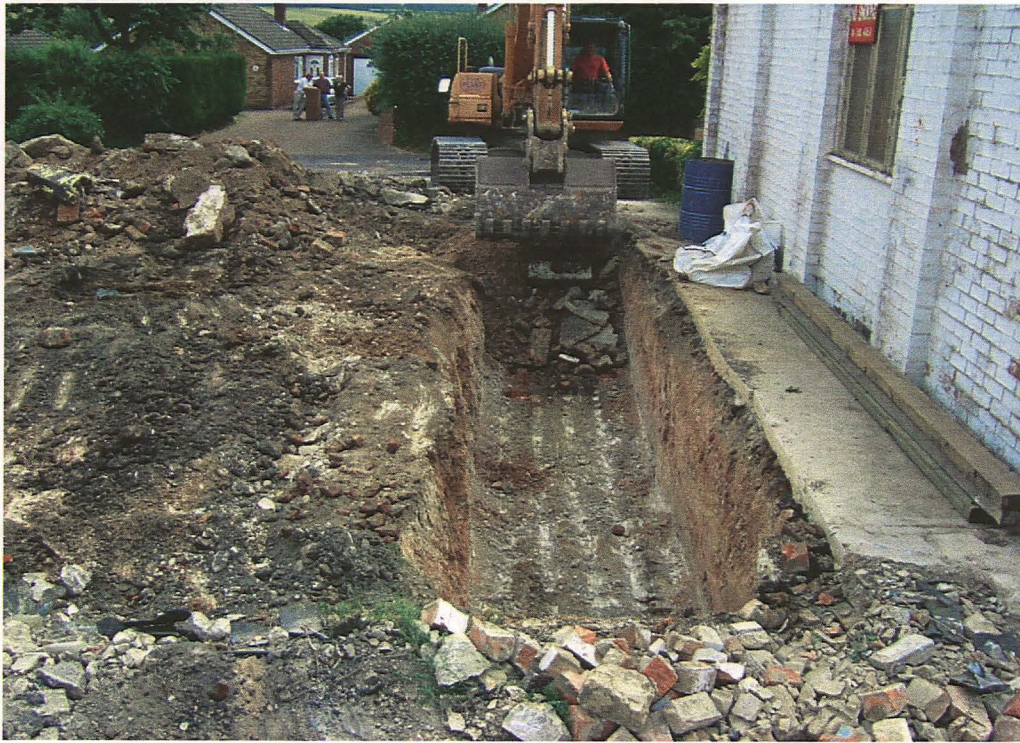
Plate 23: Shot of rectangular brick-lined pit during excavation; looking south
