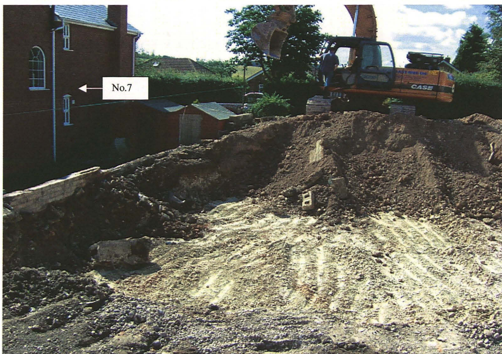
Plate 18: View across former warehouse structure following machine excavation; looking south.
