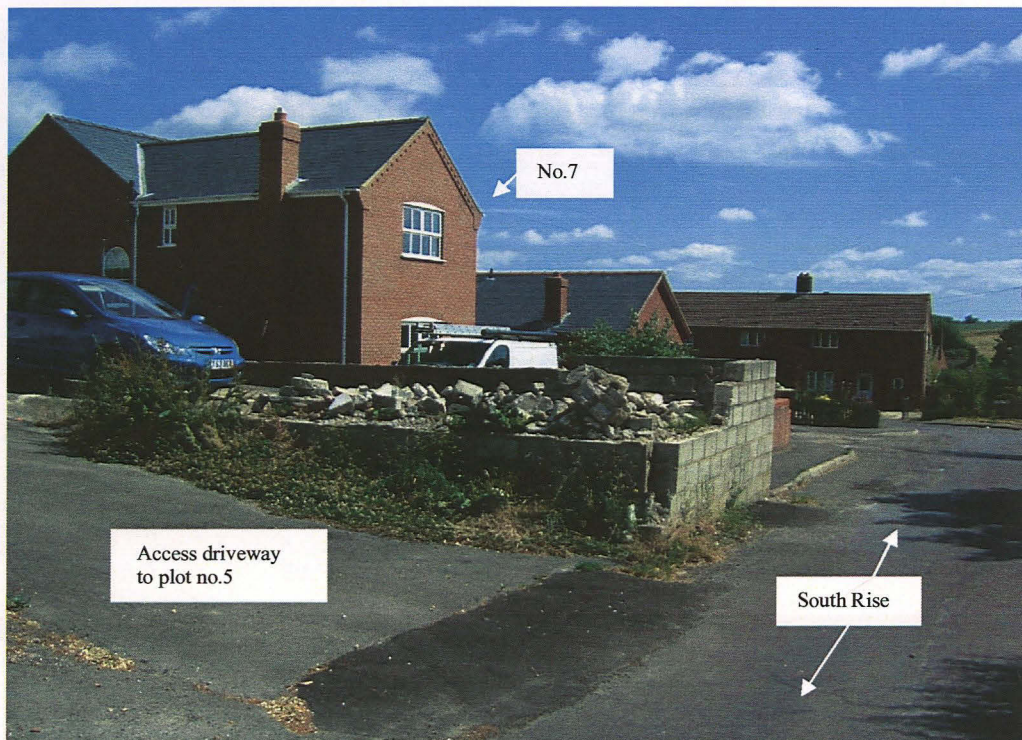
Plate 1: Tarmacked access driveway leading off South Rise road to plot no.5, looking northeast. The shot also features the raised concrete area behind which stands no.7 South Rise.
