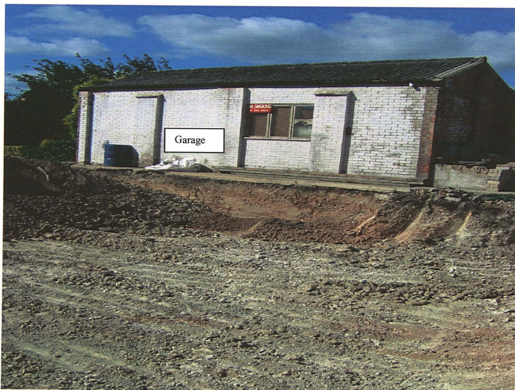
Plate 34: Looking southwest across plot no.5 towards east side of garage wall (plot no.3). This side of the garage wall almost certainly represents the west (internal) wall of the former bus depot warehouse structure.
