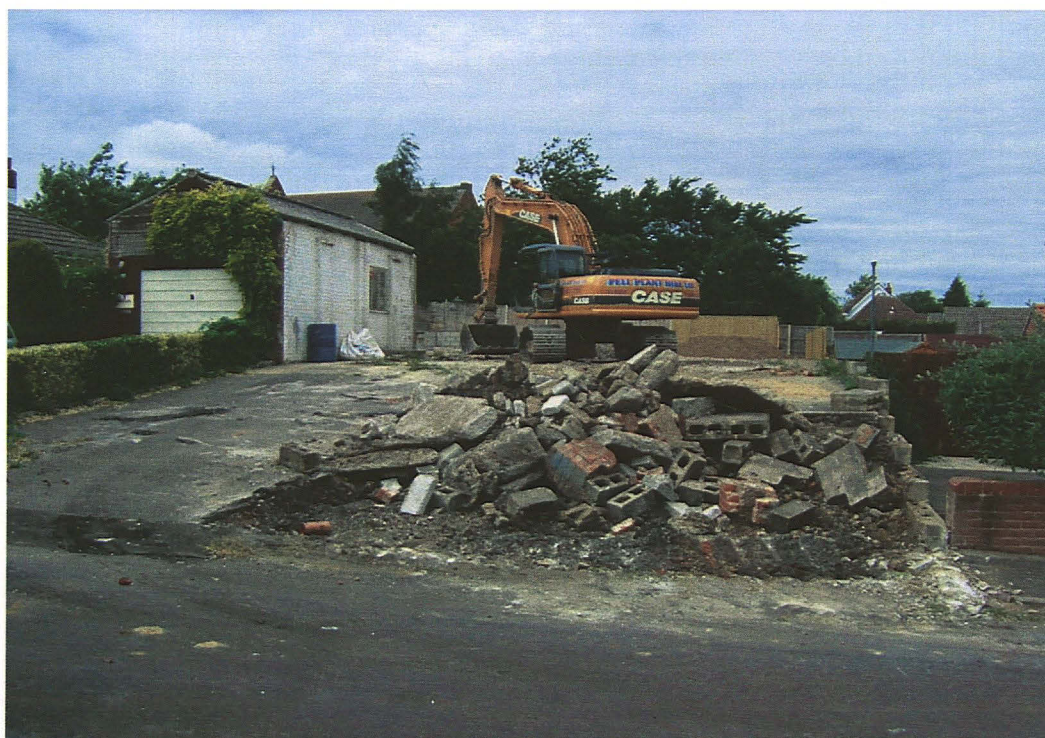
Plate 10: Rubble remains of raised concrete area following machine excavation; looking north.
