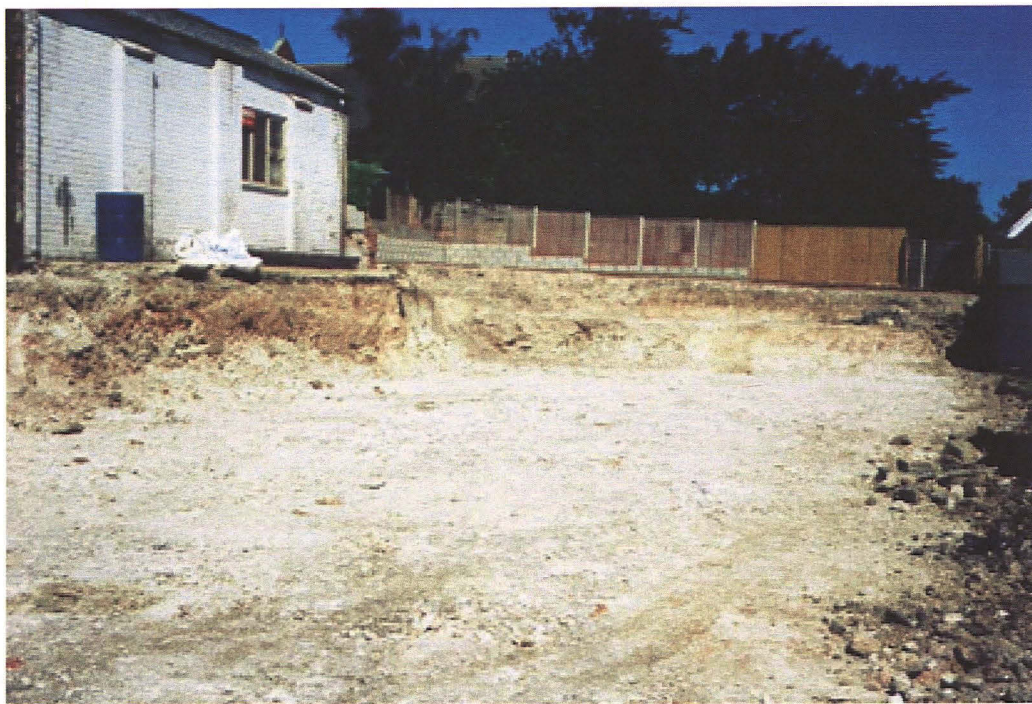
Plate 32: Plot no.5 after the completion of ground works and prior to the start of building; looking north.
