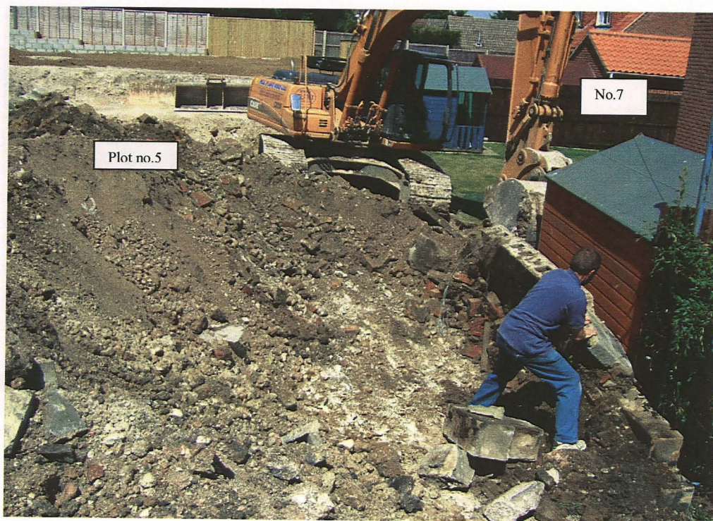
Plate 25: Dividing wall between plots nos.5 & 7 in the process of being demolished during ground works; looking north.
