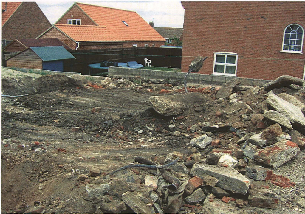
Plate 15: View across former warehouse structure following the removal of the concrete floor surface and excavation through underlying rubble; looking northeast.
