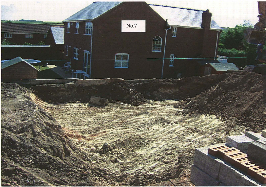
Plate 19: View across former warehouse structure following machine excavation showing the underlying chalk; looking east.
