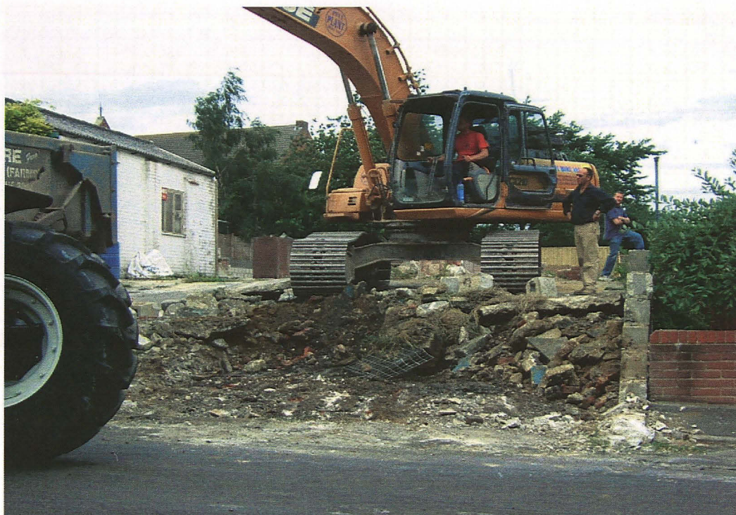
Plate 9: Levelling of raised concrete area during ground works; looking north.
