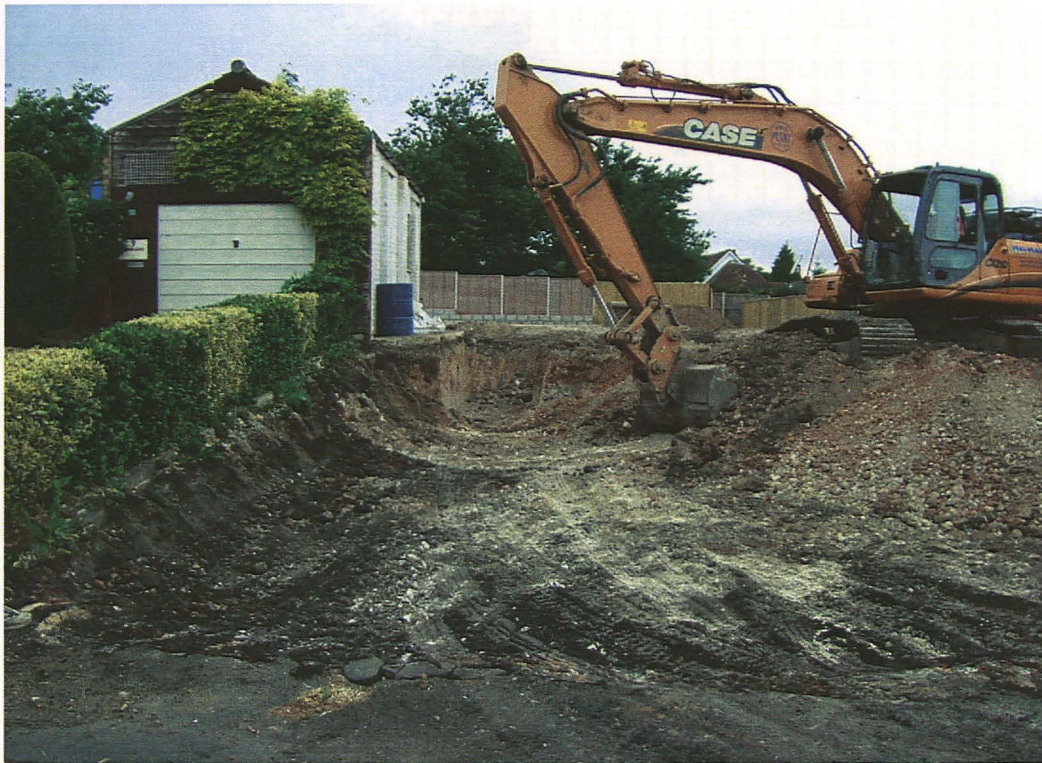
Plate 7: Entrance driveway to plot no.5 following machine excavation and removal of tarmac and underlying rubble hardcore; looking north.
