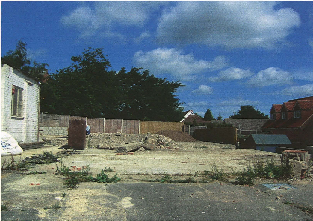
Plate 11: Featuring junction of driveway tarmac and concrete floor belonging to the former warehouse structure prior to ground works; looking north.
