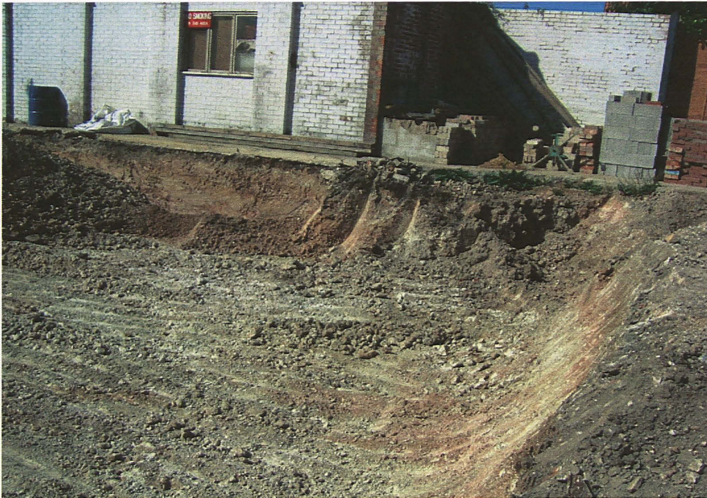
Plate 17: Looking towards the garage belonging to no.3, South Rise, and across the former location of the warehouse structure following machine excavation; looking south west.
