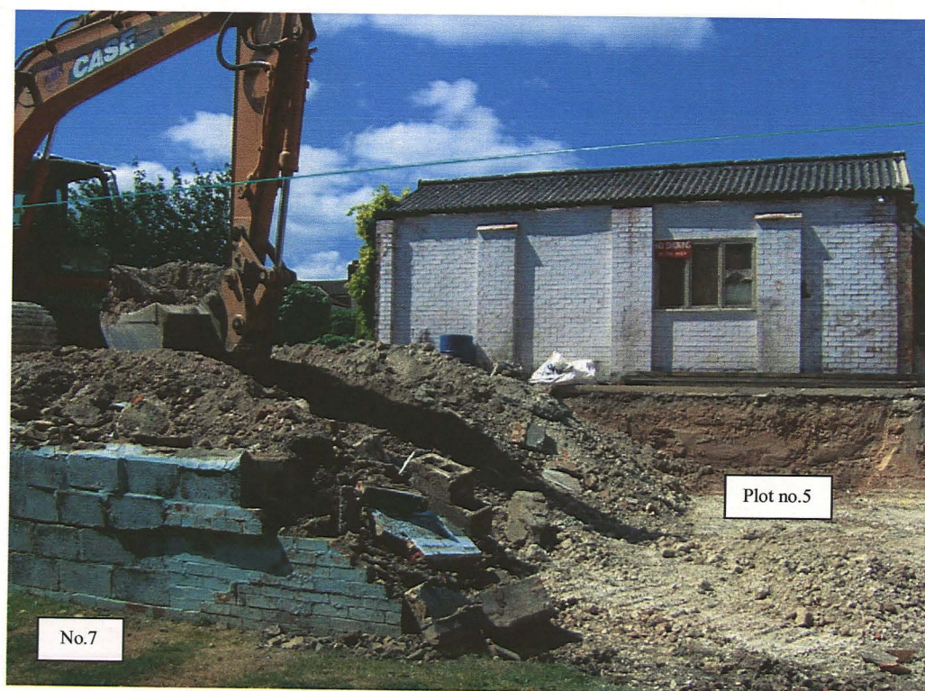
Plate 26: Concrete and brick boundary wall dividing plots nos.7 & 5 during demolition; looking west from plot no.7.
