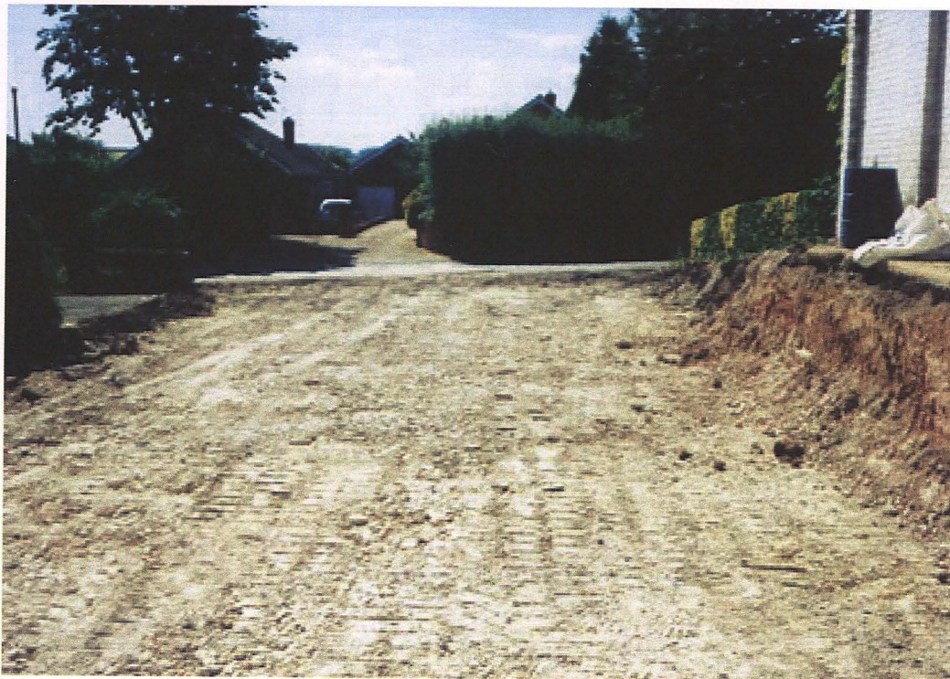
Plate 33: Plot no.5 after the completion of ground works and prior to the start of building; looking south.
