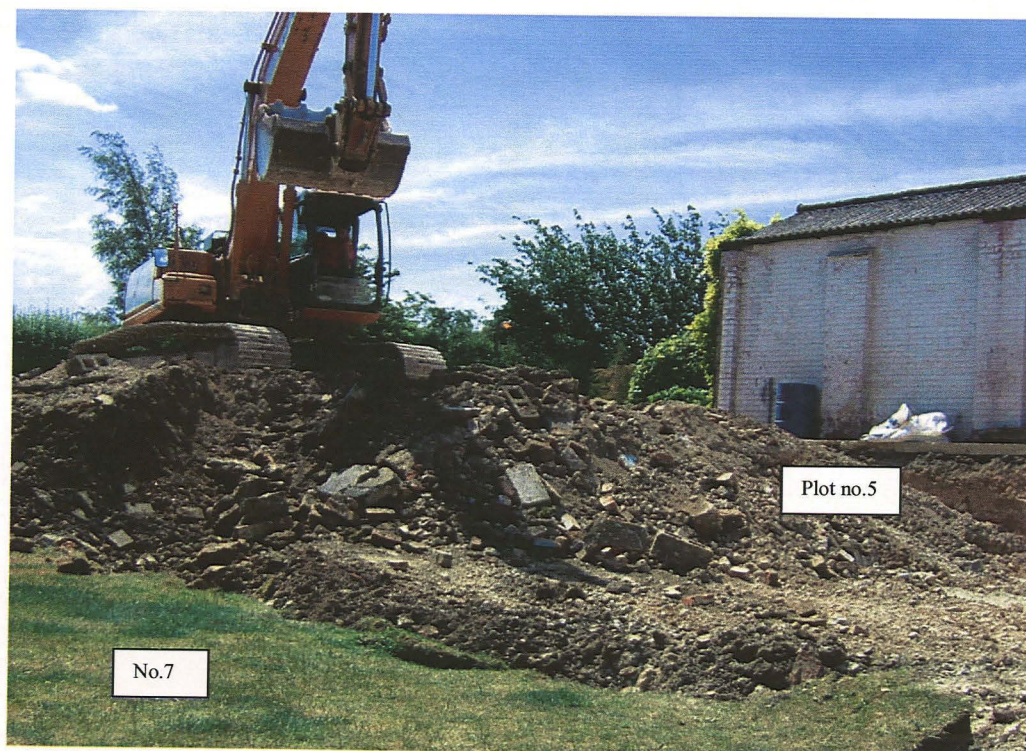
Plate 28: Looking southwest towards plot no.5 from plot no.7 during ground works, following the demolition of the dividing wall.
