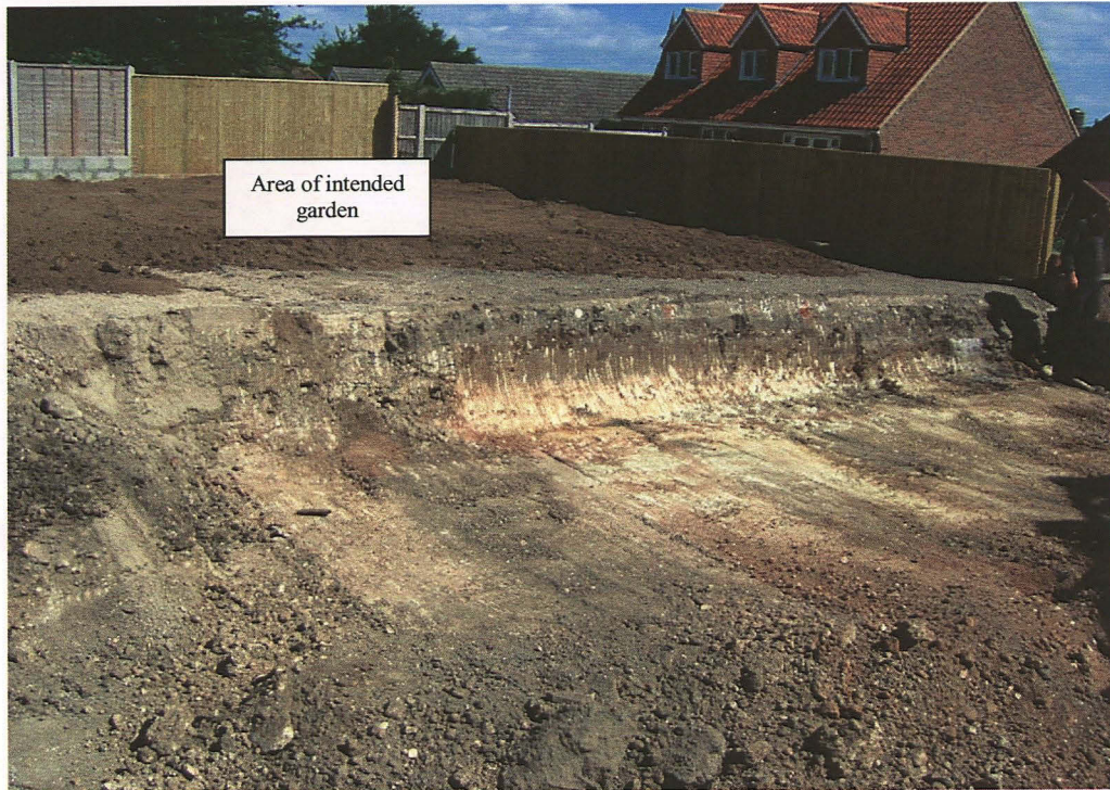
Plate 31: The north end of plot no.5 following ground works; looking northeast. Note the relatively undisturbed area of intended garden at the rear of the Plot, which features an imported layer of topsoil.
