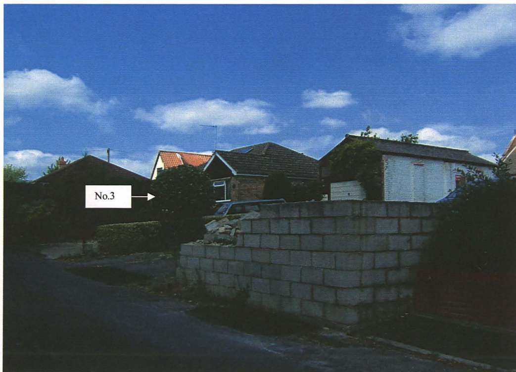
Plate 8: View from South Rise road (looking northwest) of the concrete raised area and remains of supporting breeze block walling. (The bungalow and garage building belonging to no.3, South Rise, lie in the background).
