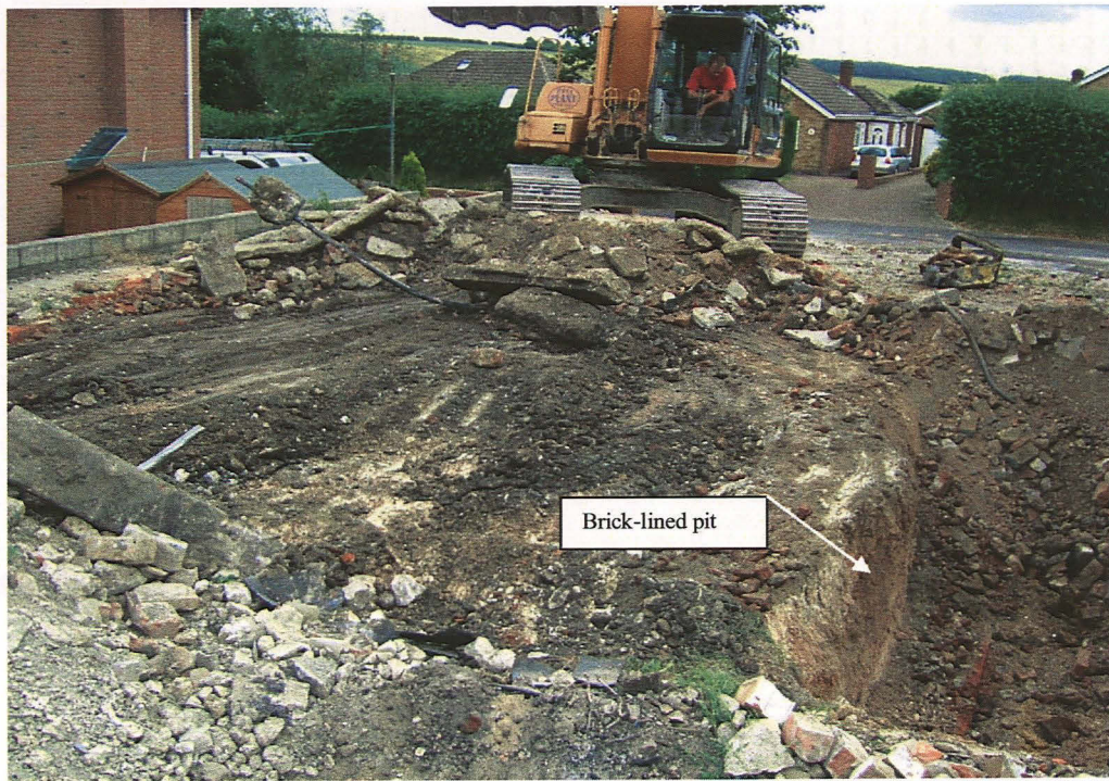
Plate 21: View across partially excavated former warehouse structure featuring the brick-lined pit to the right of the shot; looking south.
