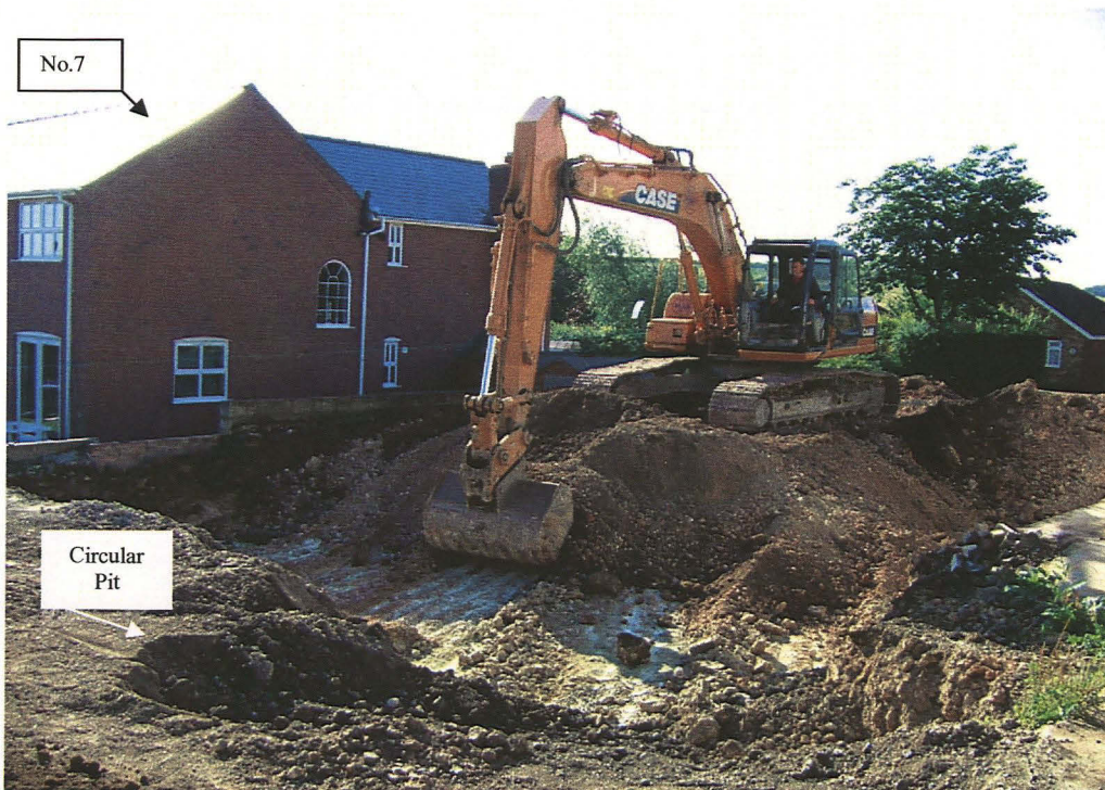
Plate 24: View across former warehouse structure during machine excavation showing partially excavated circular pit (front of shot); looking southeast.
