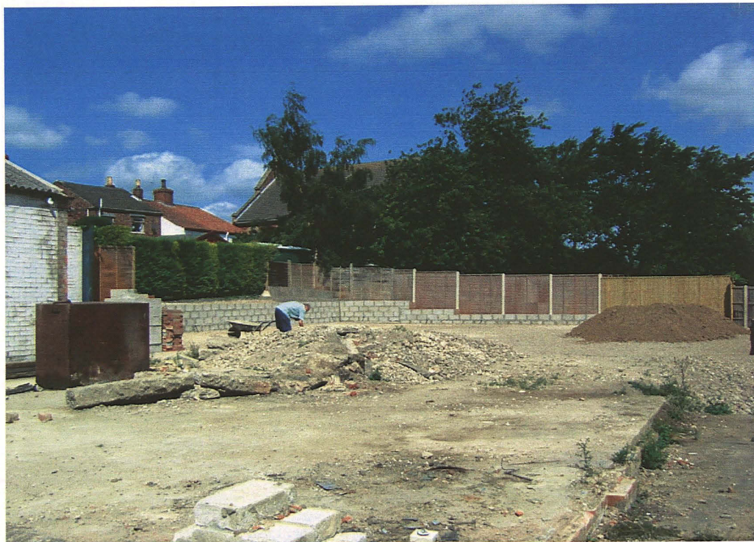
Plate 6: View across plot no.5, looking northwest, prior to the start of ground works.
