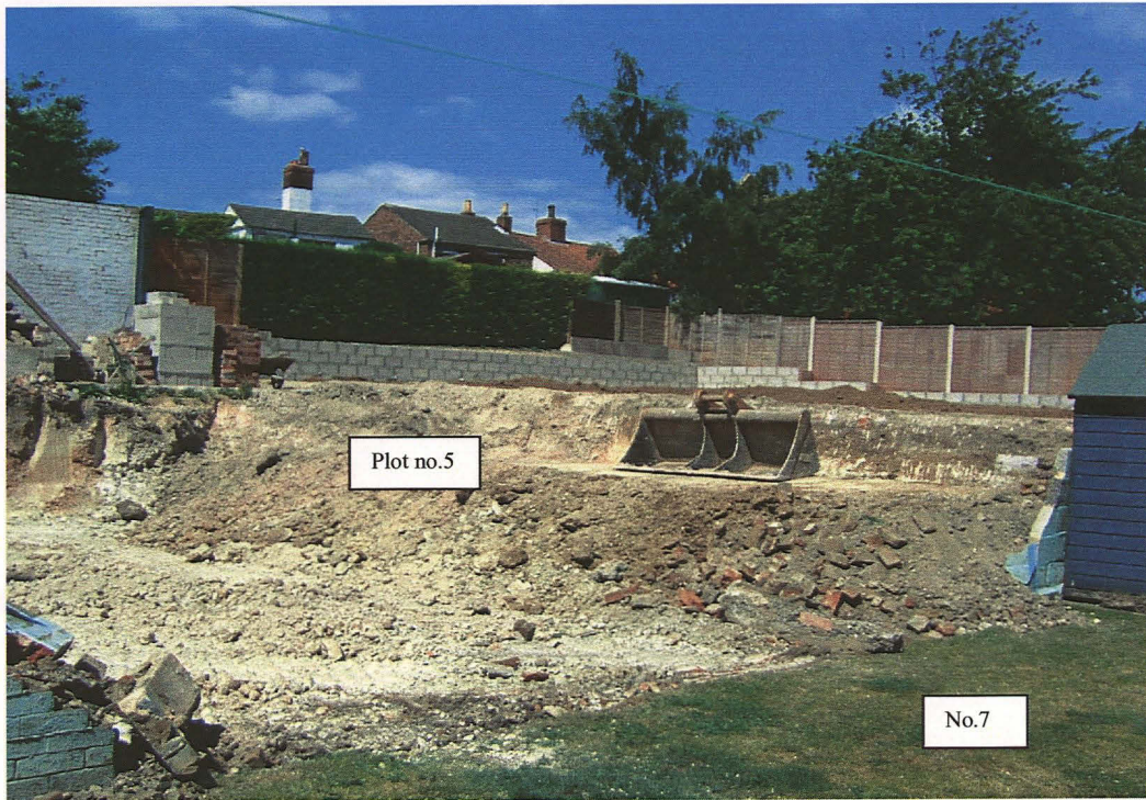
Plate 29: Looking northwest towards plot no.5 from plot no.7 during ground works, following the demolition of the dividing wall. Note the similar ground level of each plot following the excavation and levelling of plot no.5.
