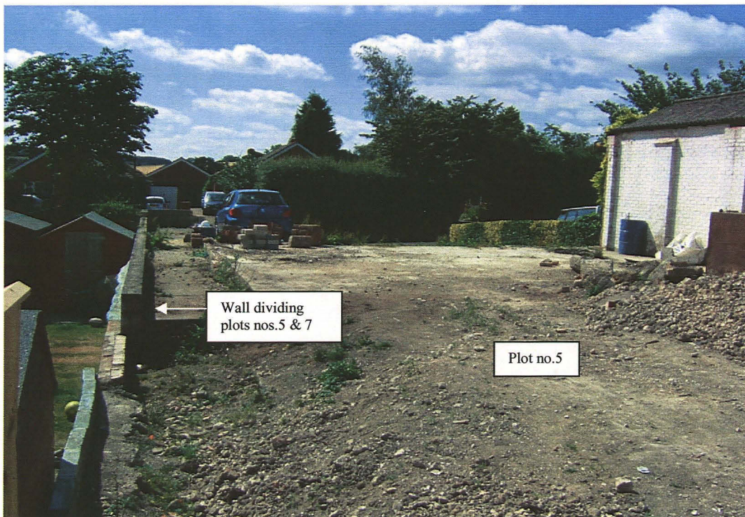
Plate 14: View across plot no.5 prior to ground works, looking south. The wall dividing plot no.5 and plot no.7 is clearly visible to the left of the shot.
