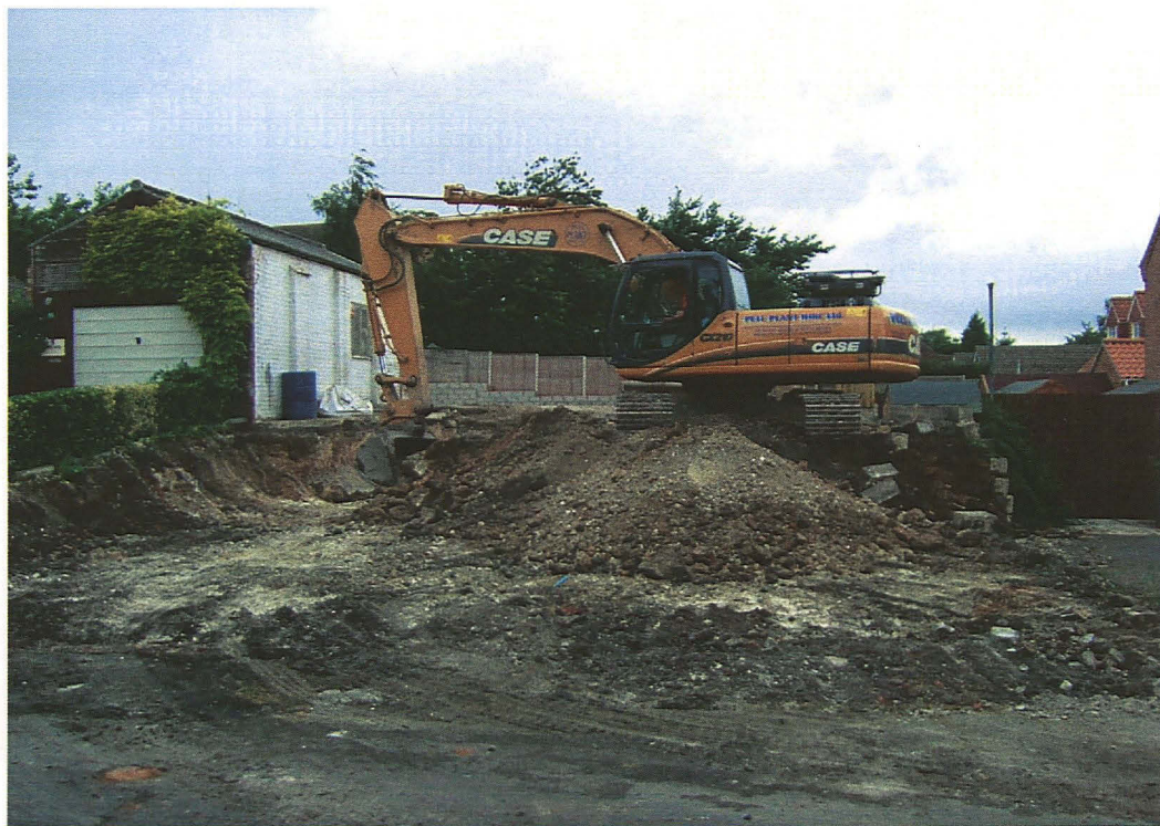
Plate 30: View across plot no.5 from South Rise road during ground works; looking north.
