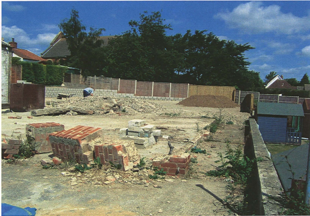
Plate 13: View across remains of warehouse structure (looking north), featuring demolished sections of warehouse brickwork.
