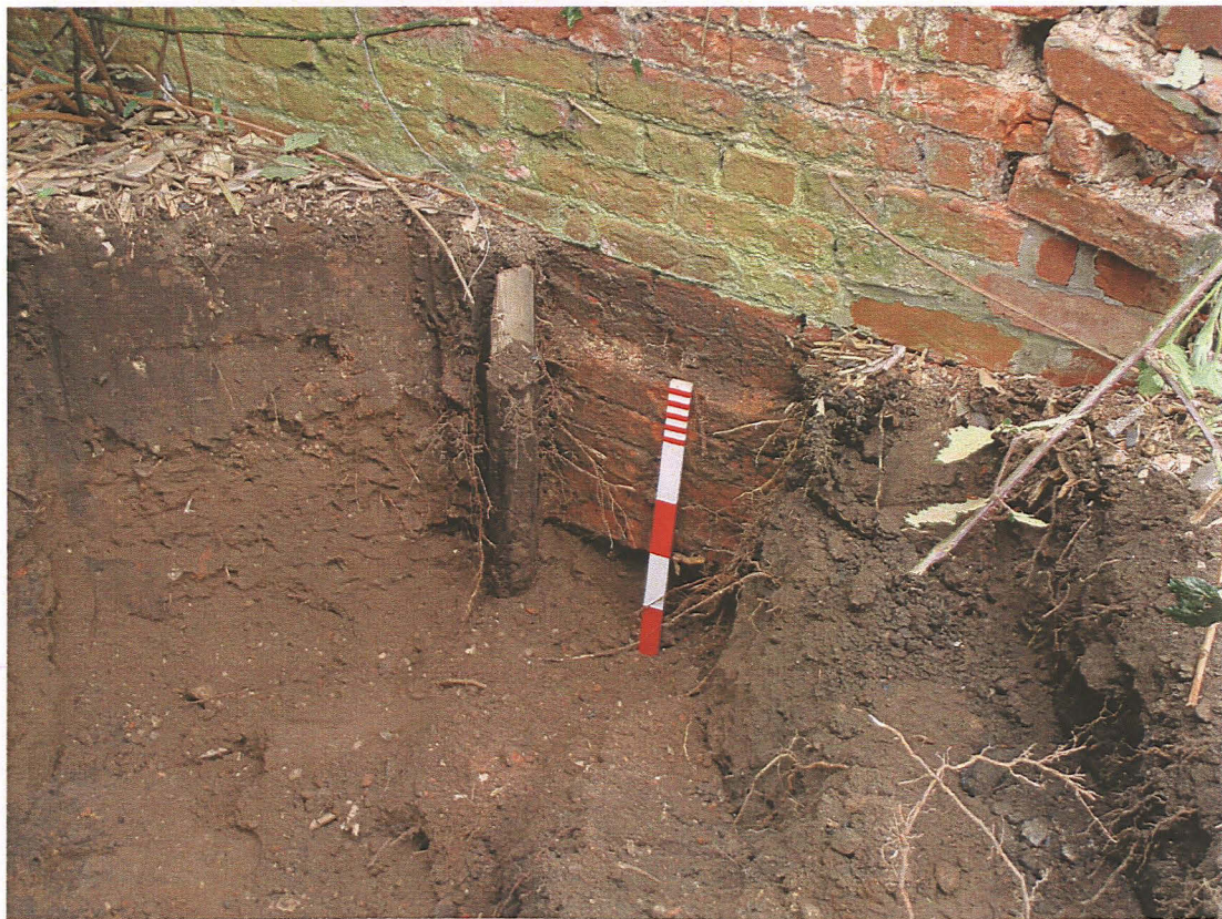
Pl. 10 Test Pit 1. Foundations of farm building. Scale 0.50m
