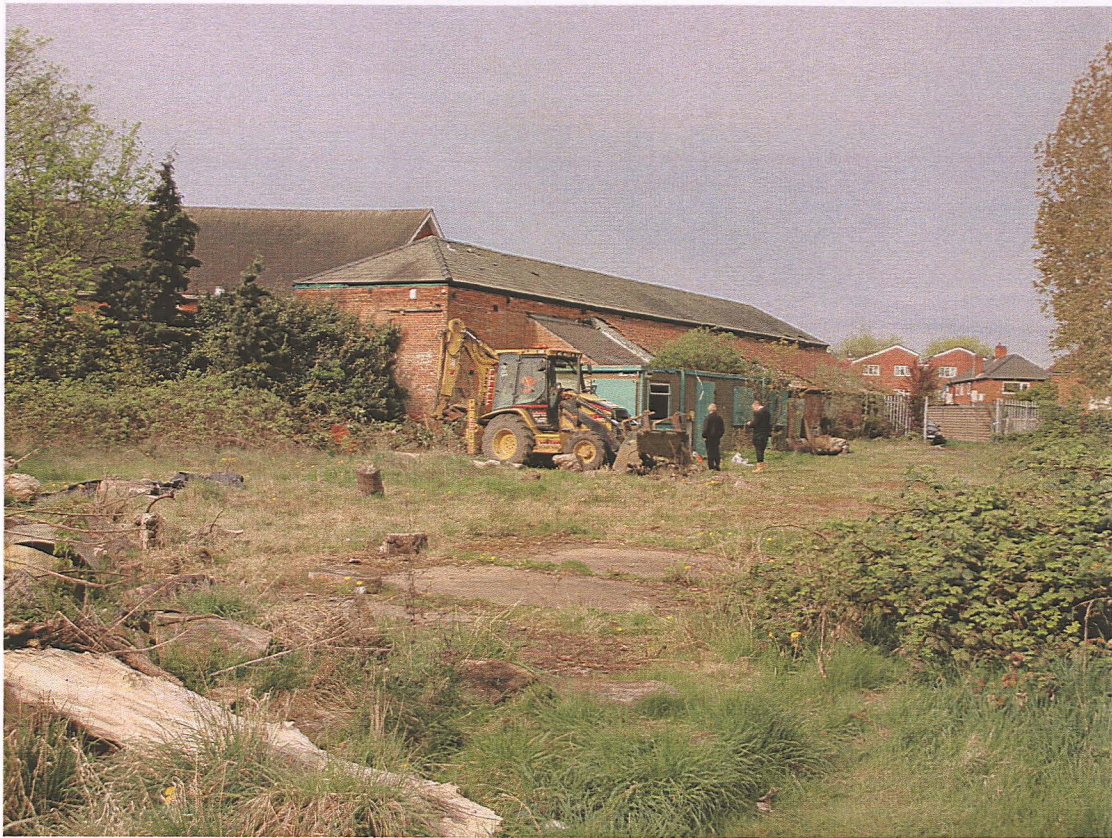
Pl. 4 General view looking west showing farm building and entrance to site
