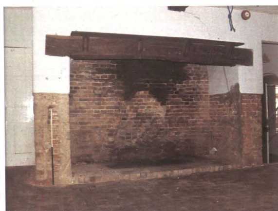
Plate 7 Room G11, fireplace with east side reconstructed
