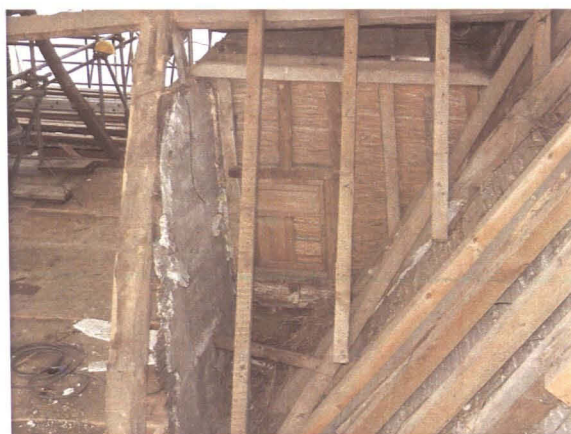
Plate 18 Eastern hatch with some panels in situ
