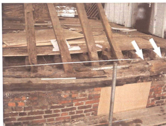
Plate 16 Wall plate in central section with the trenching of original rafters
