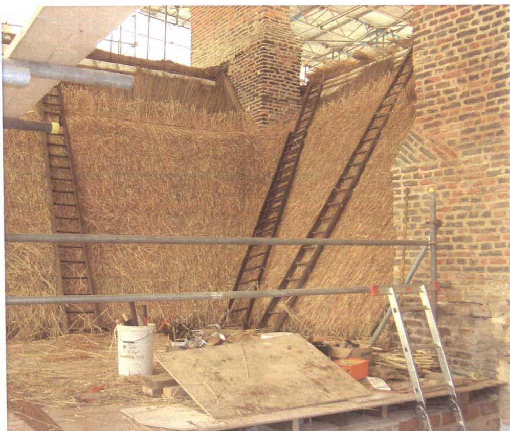
Plate 14: Re-thatching using new long straw.
