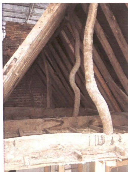
Plate 20 Unconverted timbers used to brace the ridge piece in the eastern wing
