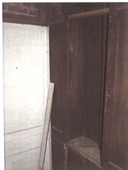
Plate 10 Closet in room F17, uncovered panelling and window shutters
