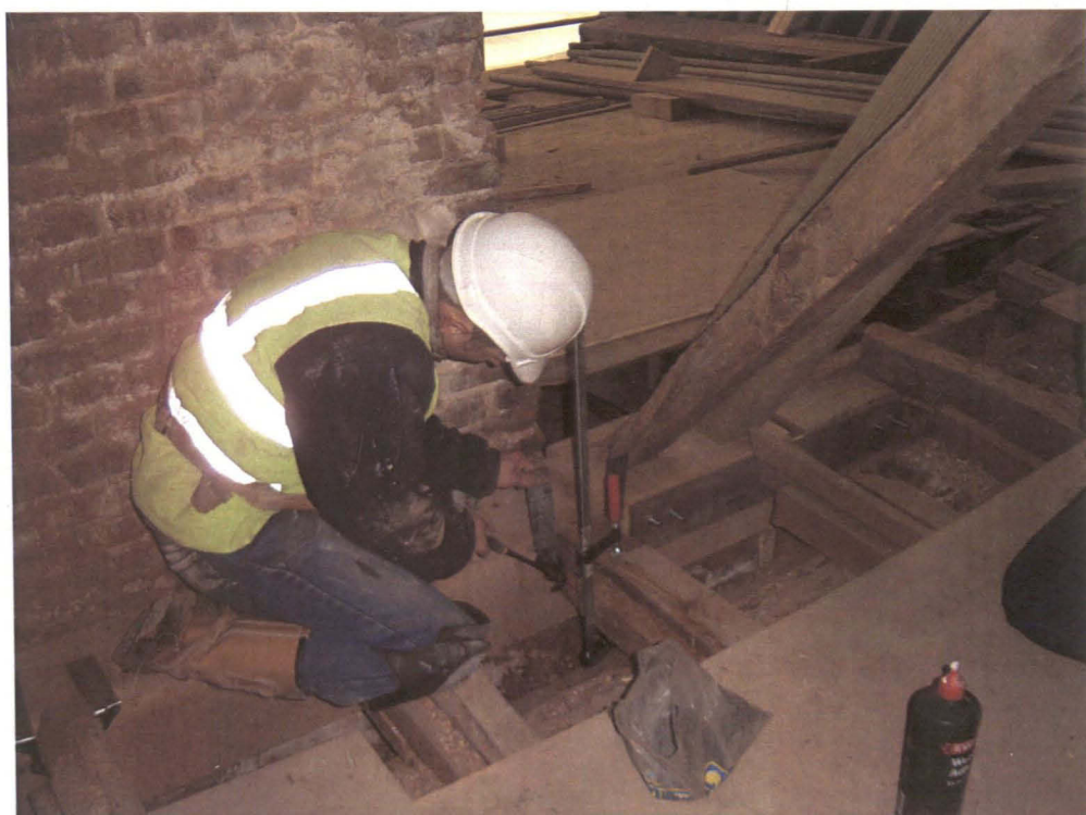
Plate 15: Repairs to oak wall-plate.
