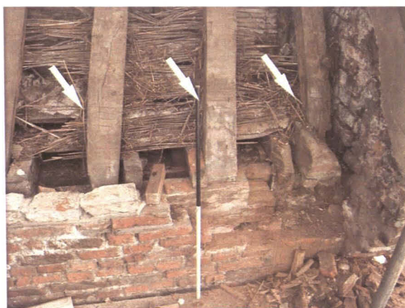
Plate 21 Common rafters labelled (from right) with a sequence of carpenters' marks
