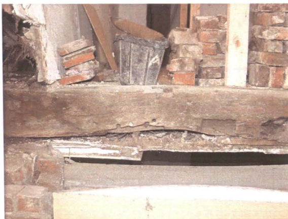
Plate 13 South gable; uncovered wall plate with lap joints
