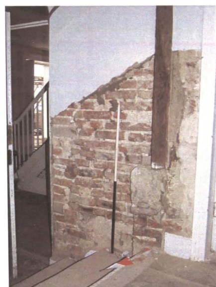
Plate 6 Room G11, in situ timber post and padstone
