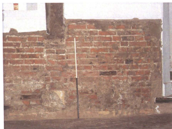
Plate 2 Room G11, shortened timber post with brick infill
