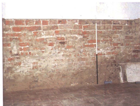
Plate 3 Room G11, scar in the wall showing the original window proportions
