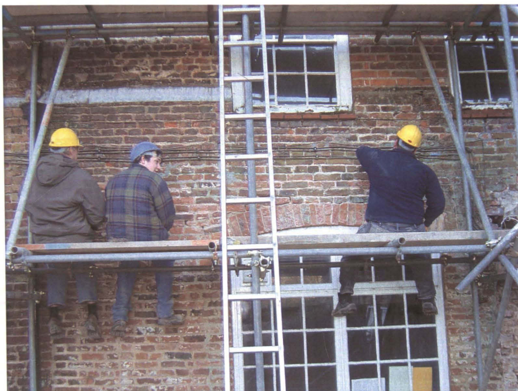
Plate 12: Repointing brickwork using pre-mixed lime putty/coarse sand.
