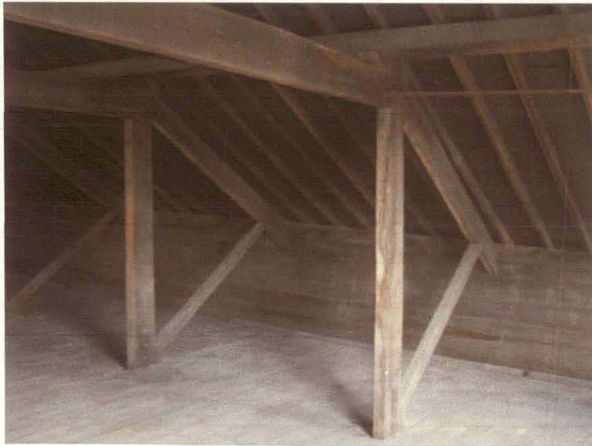
Photograph Number 13 Shows existing truss and rafters to second floor.
