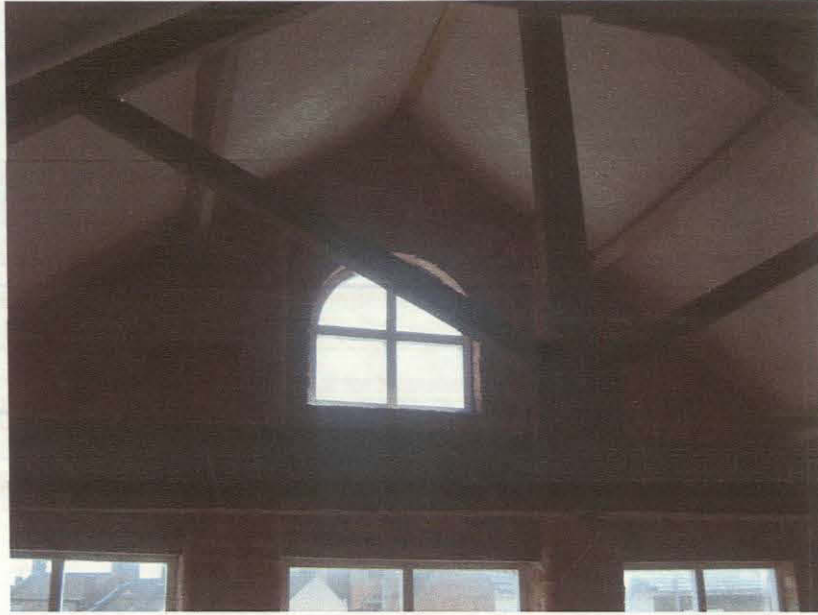
Photograph Number 12 Showing the high level window New Aluminium windows to be installed in all openings and window to be retained in this development. Window will provide light to living/kitchen areas.
