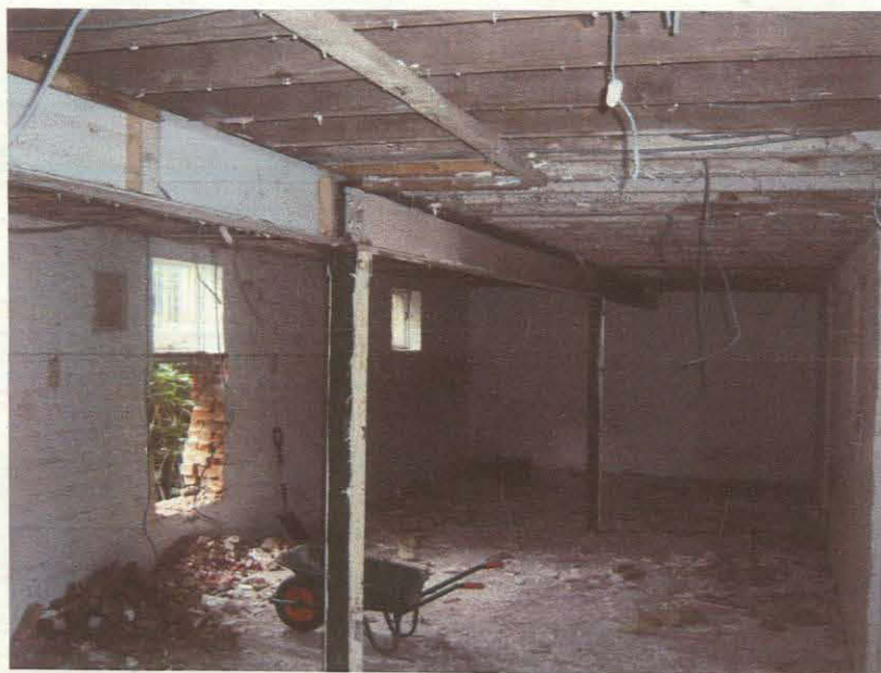
Photograph Number 4 Ground floor of 3 storey warehouse with steelwork and timber floor joists exposed
