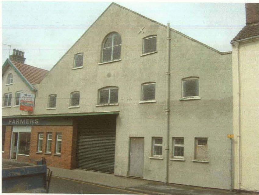
Front Elevation of Three Storey section.
