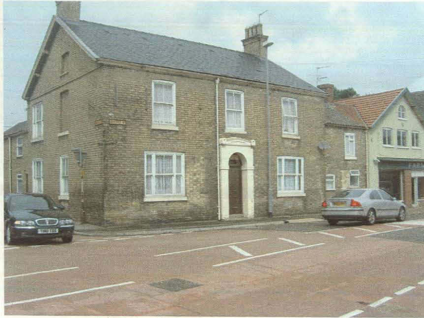
Adjoining Properties on Oxford Street
