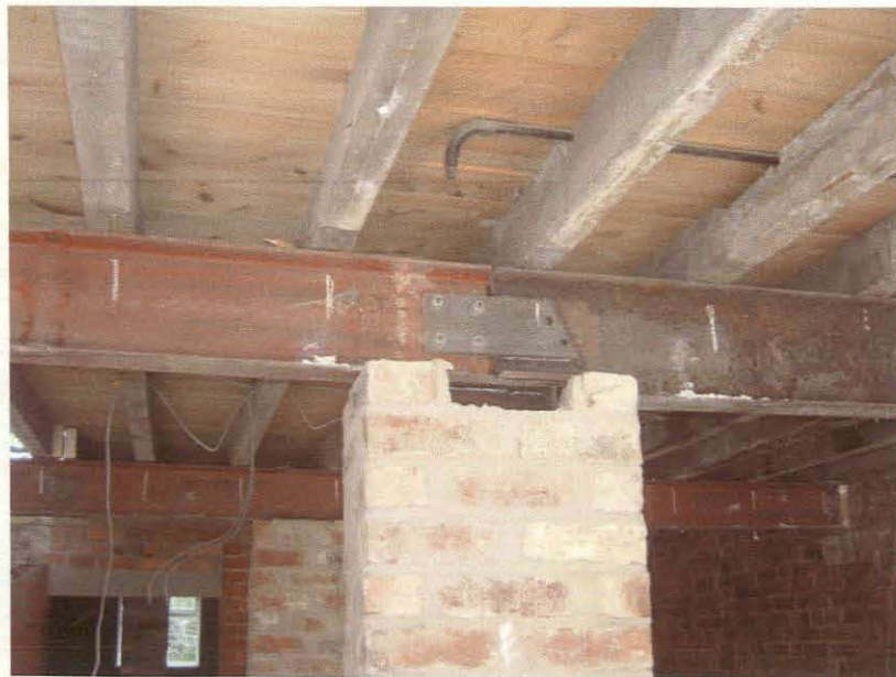
Photograph Number 2 Joint in steel beams at stanchions Note joints in timber above line of steelwork. The staining on the timber suggests that the original support structure was not on the same line. Also note slight difference in depth of steel and the inconsistency of jointing, which could suggest that these beams were replacing originally installed timber beams. Note also that the
