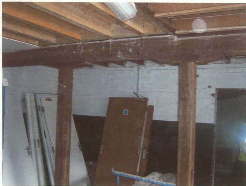
Photograph Number 6 As above. Note amendments to floor joists and the addition of steelwork to provide opening for roller shutter during former occupancies.
