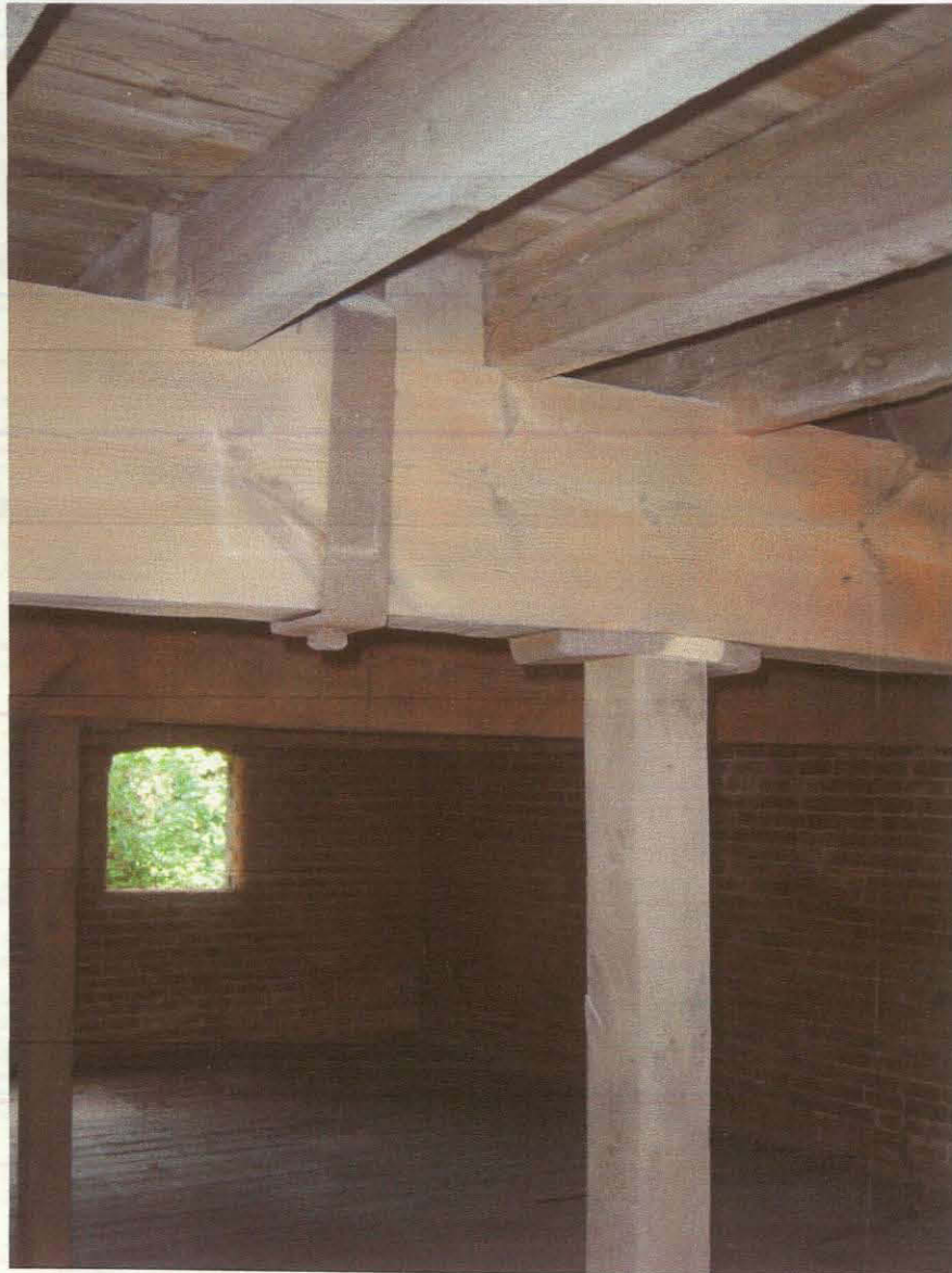
Photograph Number 9 Shows the connection between the oak stanchions to the bottom chord of the truss. Also shows the steel strapping connecting bottom chord to the truss posts.
