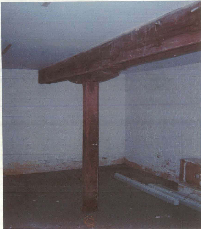
Photograph Number 5 Timber stanchion at ground floor To be retained within new development. Stanchion appears to be original structure.
