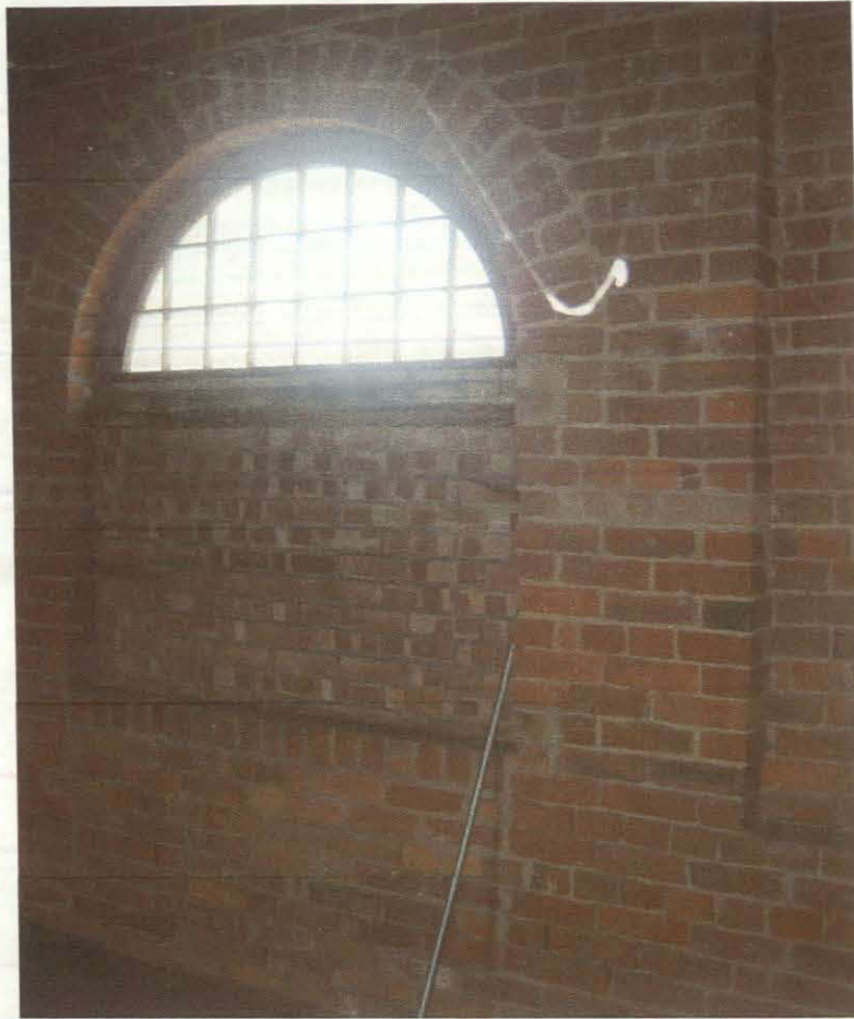
Photograph Number 16 Shows existing openings on rear elevation. Window openings to be reformed to existing sill level in this development.
