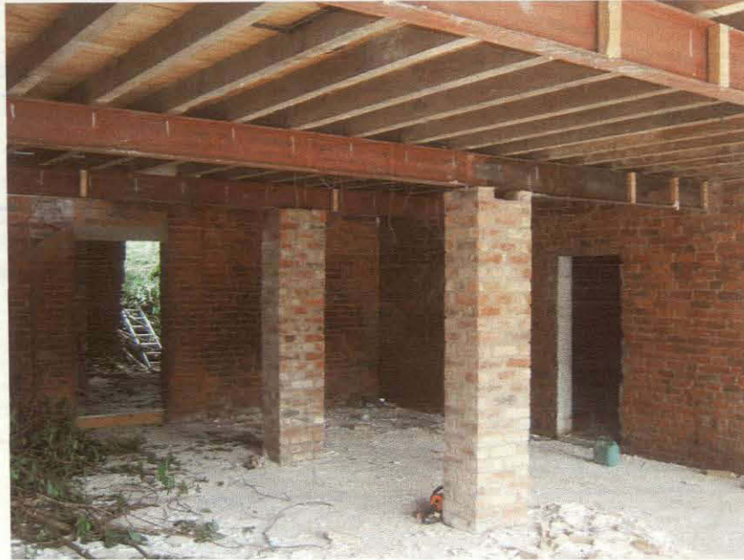
Photograph Number 1 Ground floor of retail unit showing steel support to existing floor joists Steelwork stamped Caledonian Steelwork Company Brickwork pillars hide further steel stanchions
