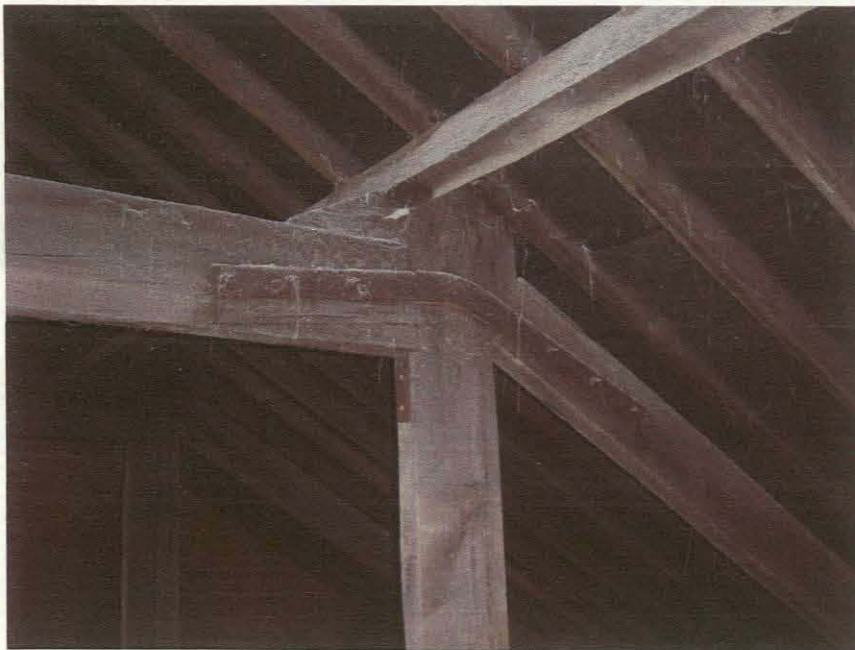
Photograph Number 15 Shows junction between truss and purlins at second floor level.
