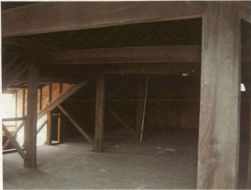
Photograph Number 14 Shows trusses at second floor and the exiting dormer and stair well. Trusses to be retained and dormer modified in height only to provide additional headroom.
