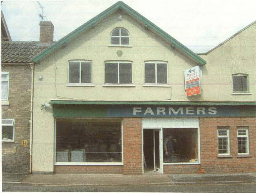
Front Elevation of Two Storey section. Former 'Farmers' retail unit.
