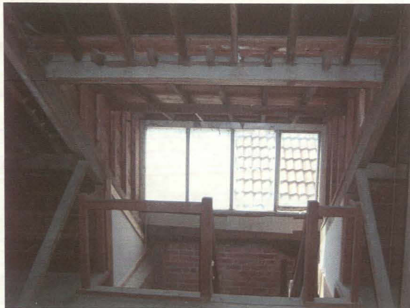
Photograph Number 17 Shows existing dormer above stair well.
