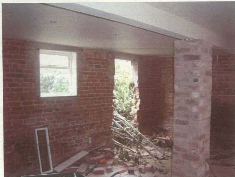
Photograph Number 3 Openings formed in existing structure during previous occupancies Note use of concrete lintels and that windows do not accord with brick coursing Steel beams and stanchions with brick cladding.
