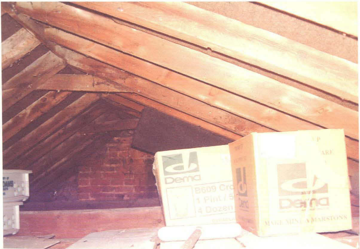
Plate 17. Replaced roof timbers.
