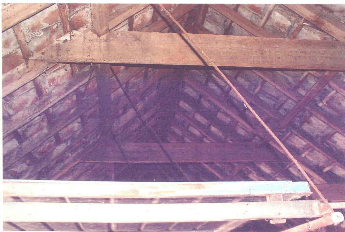
Plate 4. Showing replaced modern roof timbers in barn.
