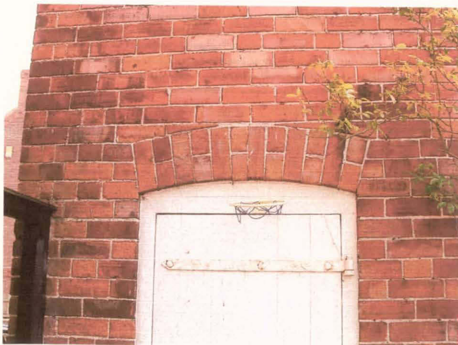
v) Detail – brick arch above West facing door
