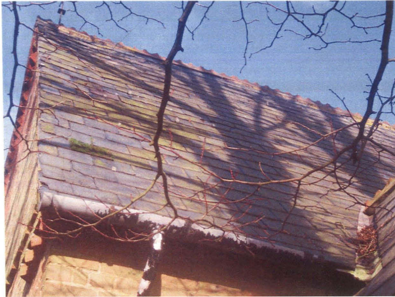
Figure 7 South nave/chancel roof covering, showing remedial tingles to slates and debris to porch valley gutter.
