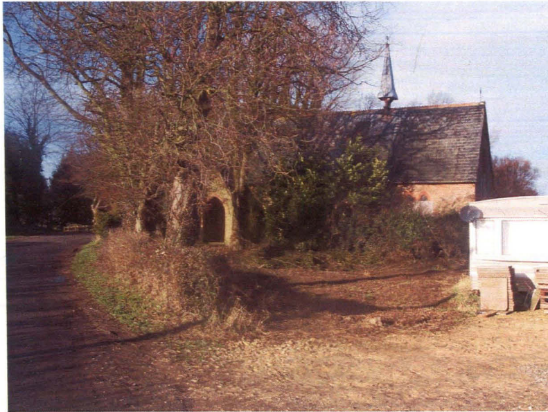
Figure 1 General view of church from south, showing highway, hedge and railing boundary, cleared ground and static caravan.
