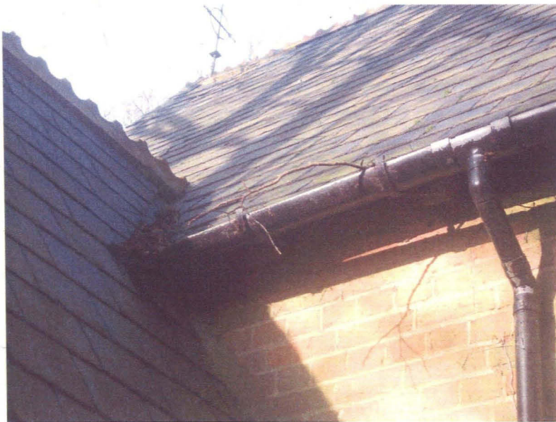
Figure 8 South nave/chancel roof covering, showing debris to porch valley gutter.
