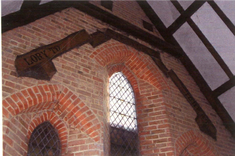
Figure 35 Chancel east wall with painted banner stating 'Glory to God in the Highest' over window (W5).
