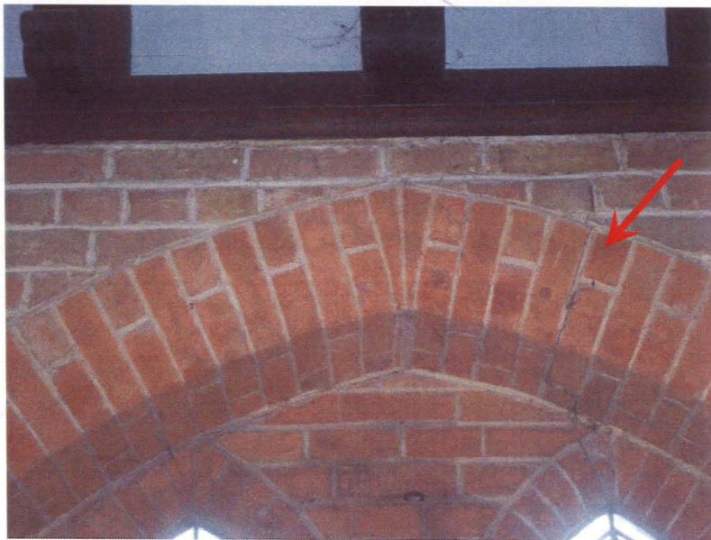
Figure 33 Chancel north wall, showing cracking over window (W1) (arrow).
