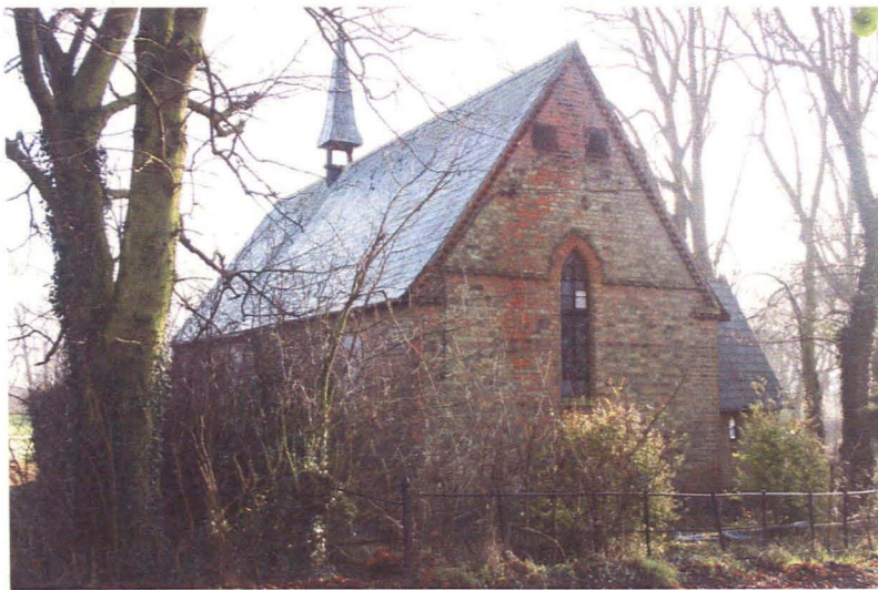
Figure 2 General view of north and west elevations, with hedge and railing boundaries and mature trees. Note absence of boarding to window (W9).
