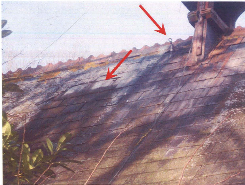
Figure 9 South nave/chancel roof covering, showing displaced slates and remedial tingles over assumed ventilator to west of flèche (lower arrow). Note lightning protection down conductor from flèche and assumed rope penetration for bell chiming (upper arrow).
