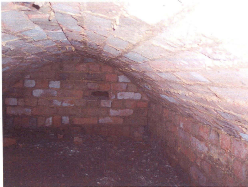
Figure 37 Chancel floor, with observed vault (see Fig. 38). Note ventilation hole to assumed eastern vault.
