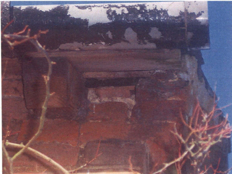
Figure 26 Upper chancel south elevation, showing gap beneath projecting eaves.
