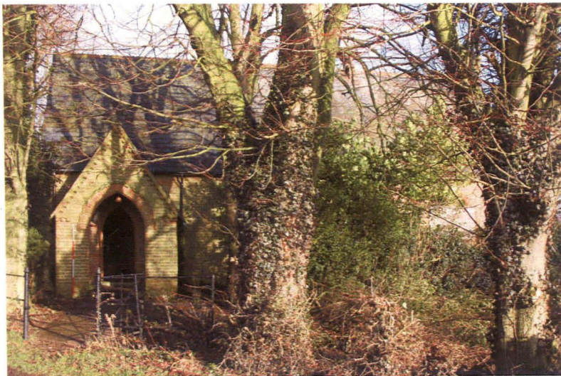
Figure 4 General view of south elevation, with path to porch and mature trees.
