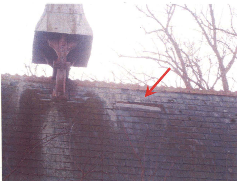
Figure 6 North nave/chancel roof covering, showing displaced slates and remedial tingles over assumed ventilator (arrow).
