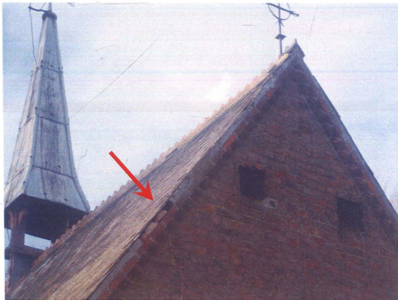
Figure 17 Upper chancel east elevation, showing damage to verge mortar (arrow) and failing mortar and/or brick displacement possibly associated with corrosion around ventilators.
