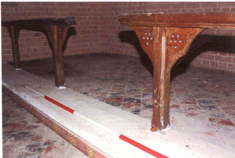
Figure 46 Altar rail with missing hinged central section, with decorative ceramic tiles to step riser and tiles to chance/sanctuary floors.
