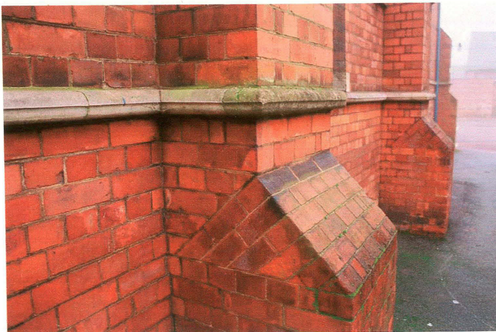
03 Brickwork buttressing and simple stone stringcourse to South elevation
