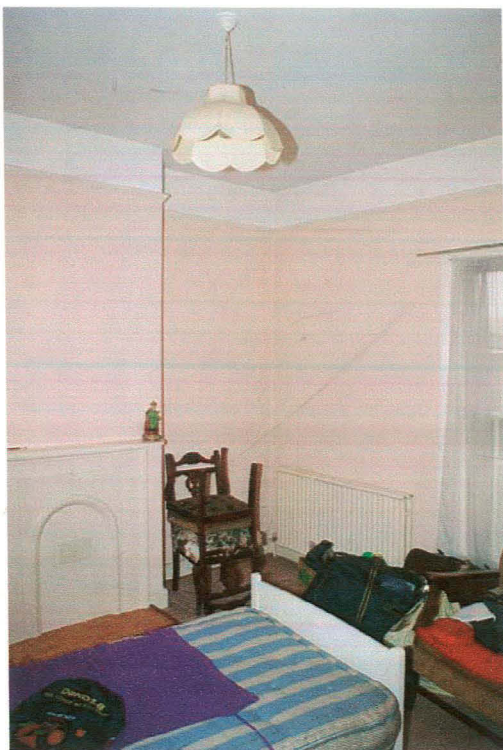
63 Priory bedroom 2 showing picture rail cast iron fire surround and simple sunk bead skirting
