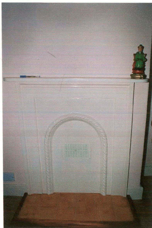
63 Priory bedroom 2 showing picture rail cast iron fire surround and simple sunk bead skirting
