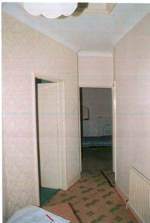
61 Priory landing showing modern chamfered architrave and skirtings and modern plaster coving to ceilings
