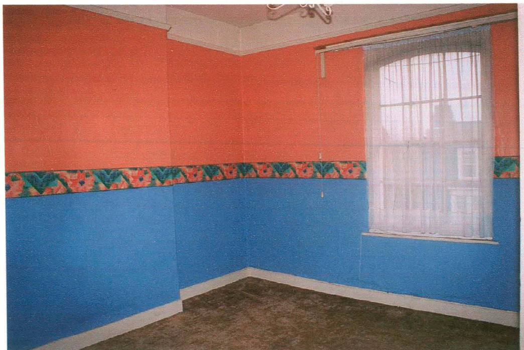
44 Bedroom 1 with picture rail intact and "6 on 6" sash window but modern chamfered skirtings
