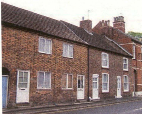
Gospeigate – erosion of traditional detailing with replacement windows and roof covering and loss of chimneystack
