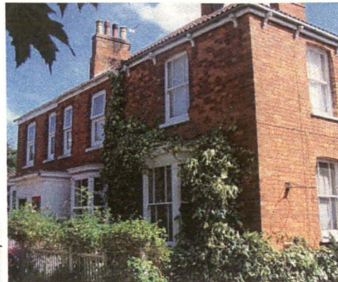
Gospeigate – erosion of traditional detailing with replacement windows and roof covering and loss of chimneystack
