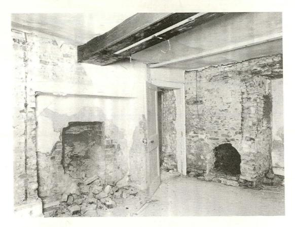
The ground floor of the formerly vaulted north bay from the south-west, showing the inserted stack and ceiling
