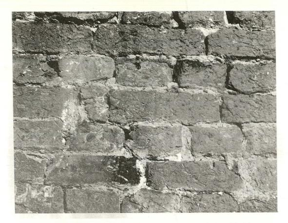
Brickwork in the vaulted bays, showing sintered and glazed bricks
