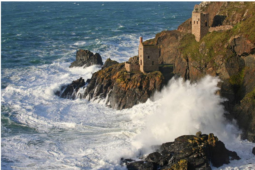
Fig 11 Botallack tin mine in Cornwall (photo Cornwall Council)
