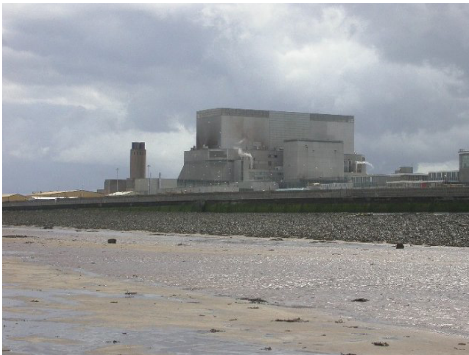
Fig 12 Hinkley Point power station, Somerset (© Copyright Robin Somes and licensed for reuse under this Creative Commons Licence )
