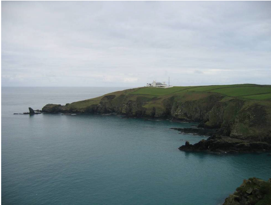
Fig 8 The Lizard lighthouse (Cornwall Council)
