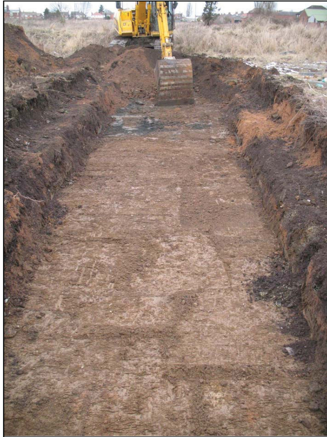
Plate 1: Working shot of Trench 3 showing sandy-clay natural; viewed facing north; 1m scale
