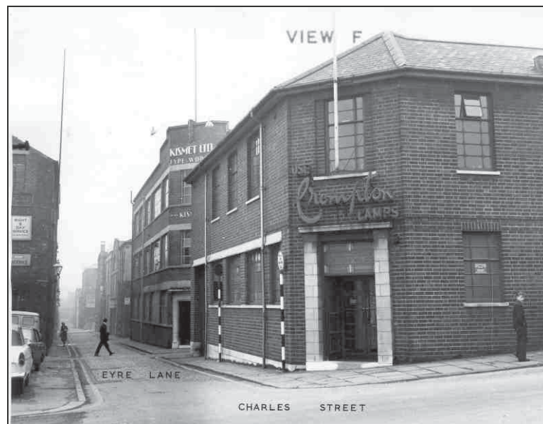
Plate 3: View of 1930s-40s extension to the Canada Works, Charles Street, in 1967, with the Eyre Street Works to the rear (© Copyright Sheffield City Council)
