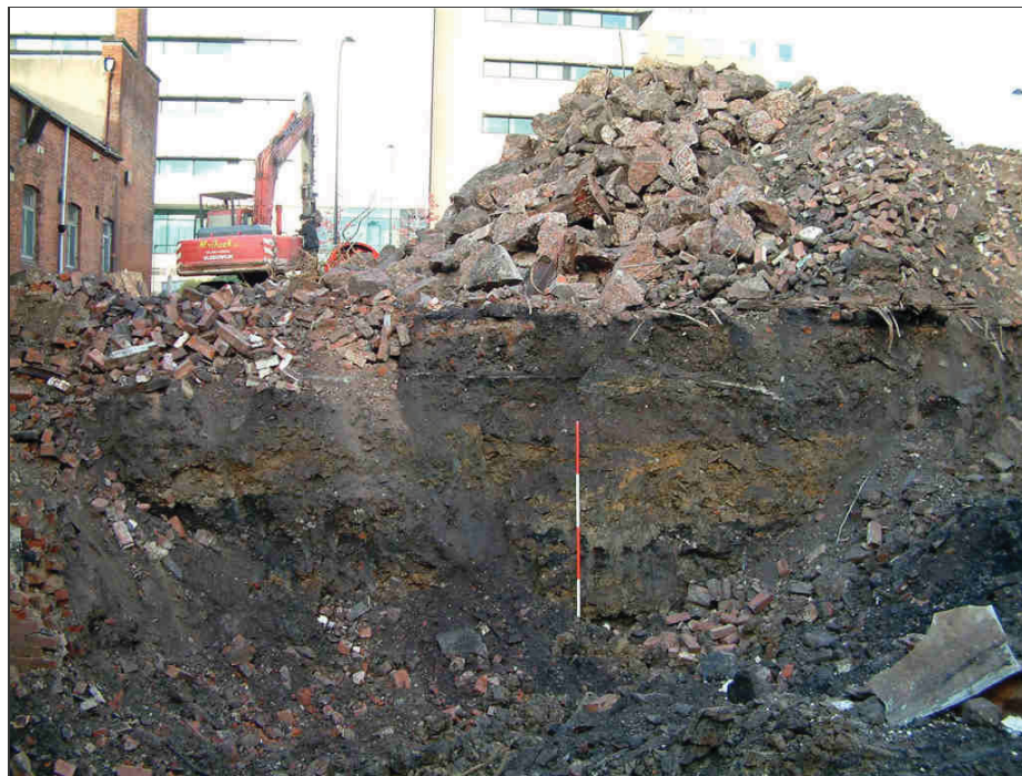
Plate 10: Section through made ground beneath Building D, viewed from the east (© Matrix Archaeology)
