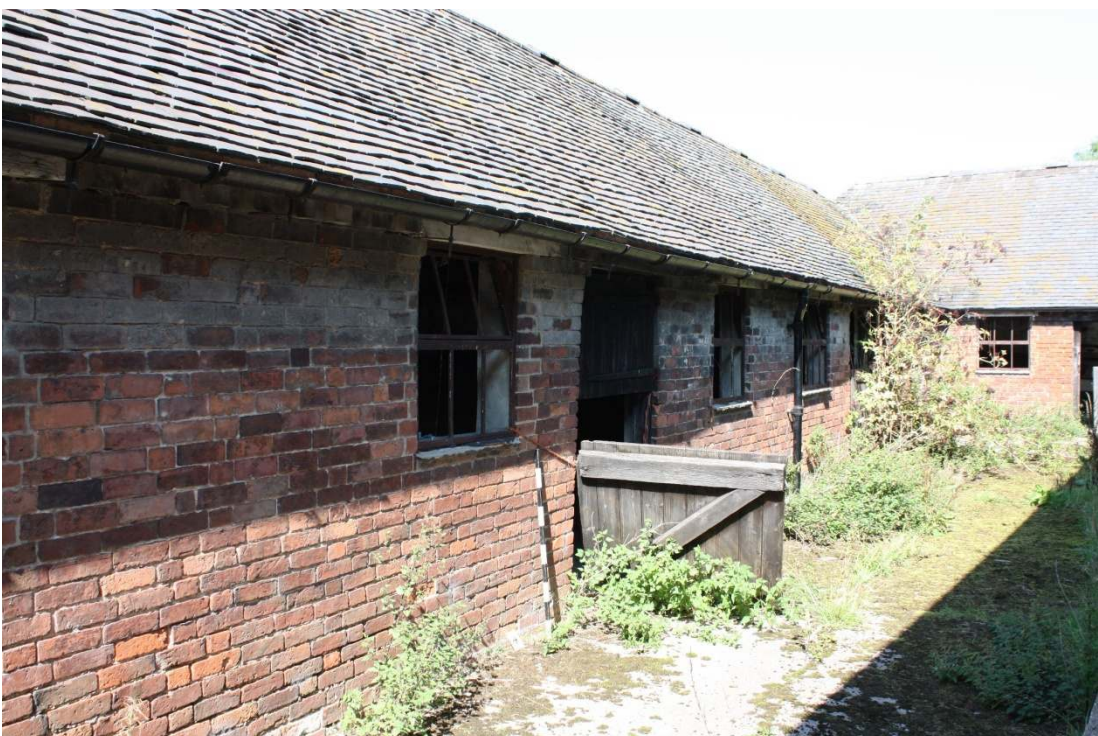
Plate 8: East face of cowshed range 1, viewed facing north
