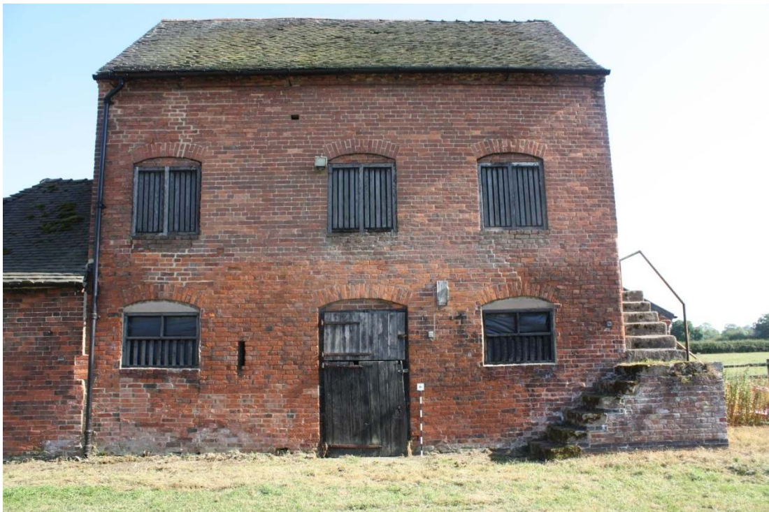
Plate 14: Northwest face of stable, viewed facing southeast
