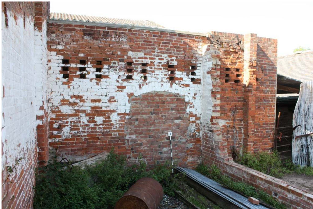
Plate 4: Part of west wall of Barn 2, viewed facing north
