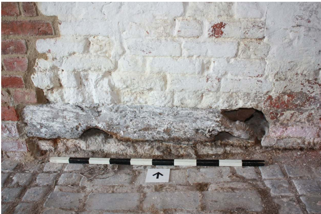
Plate 18: Reused timber plate at base of cross-wall in stable, with a possible head carved at right end, viewed facing northeast
