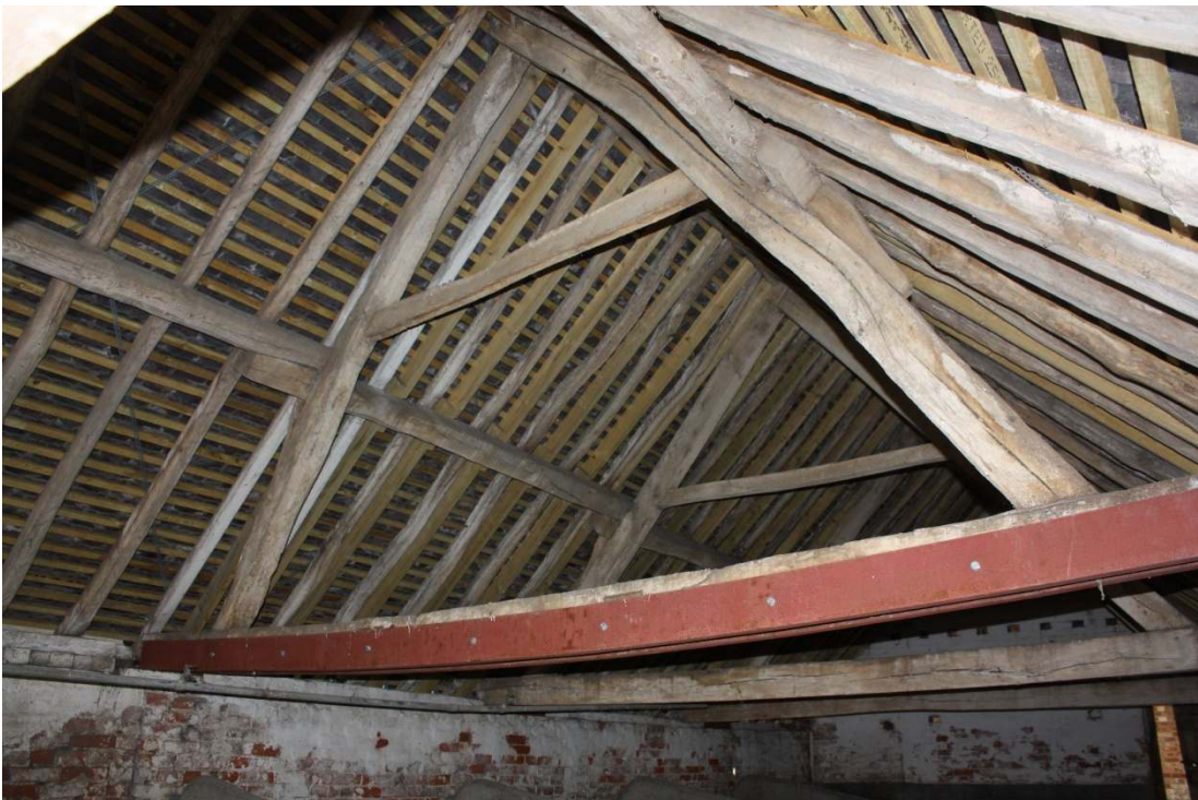
Plate 10: Plain roof trusses to east of straight joint in cowshed range 2, viewed facing east
