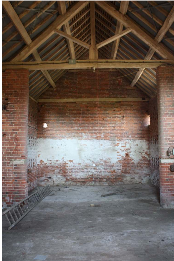
Plate 3: View along interior of barn showing spur walls, facing northeast
