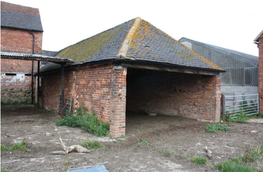
Plate 21: Open-ended shed to east of main stable, with blocked-in side, viewed facing north
