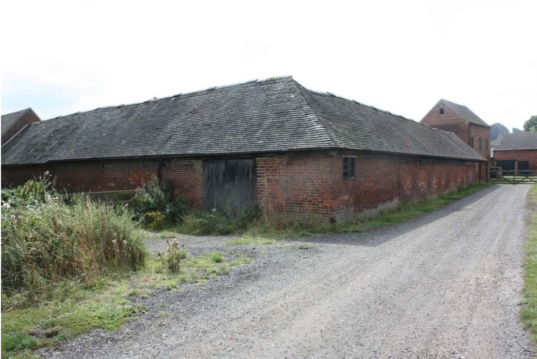
Plate 7: Northeast and northwest faces of cowsheds and barn, viewed facing south
