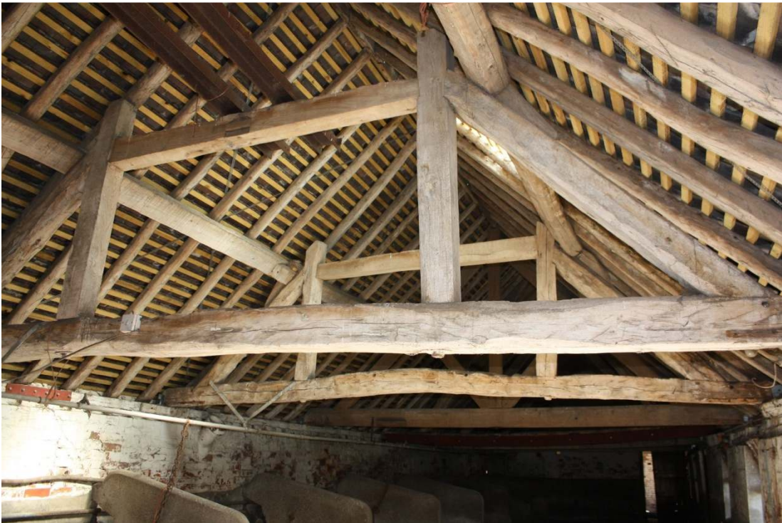
Plate 11: Queen post trusses to west of straight joint in cowshed range 2, viewed facing southeast
