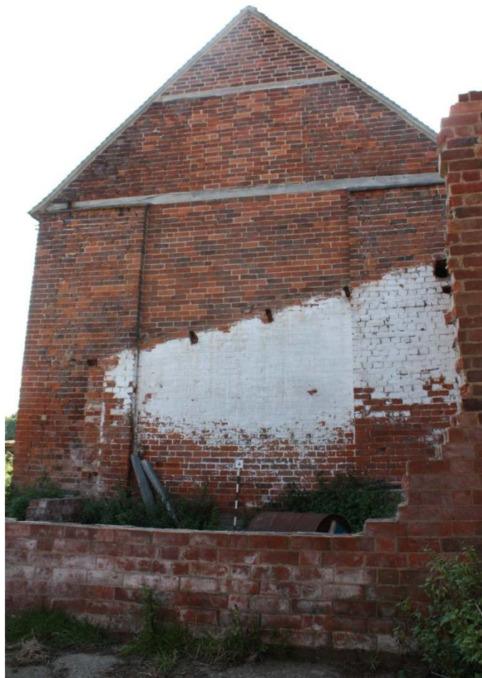
Plate 5: North face of barn showing former roof line of Barn 2, viewed facing southwest
