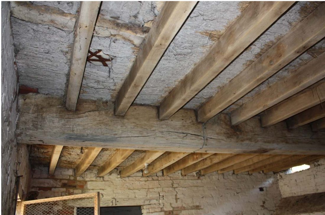
Plate 17: Chamfered beam and joists supporting first floor of stable, viewed facing northeast
