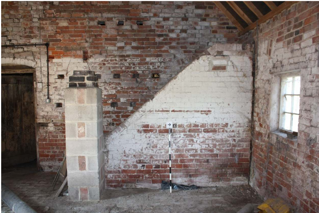
Plate 13: Redundant staircase in east end of cowshed range 2, viewed facing northwest
