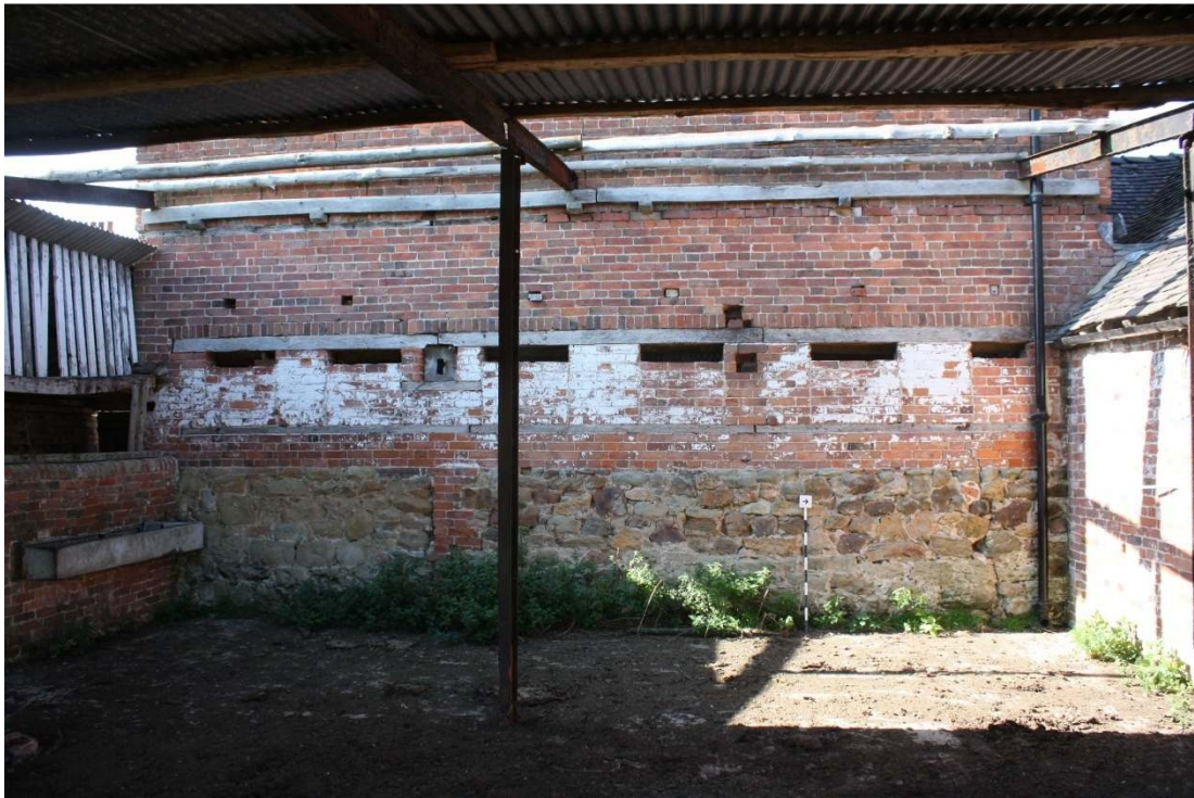
Plate 15: Southeast face of stable, showing stone wall at base, viewed facing northwest
