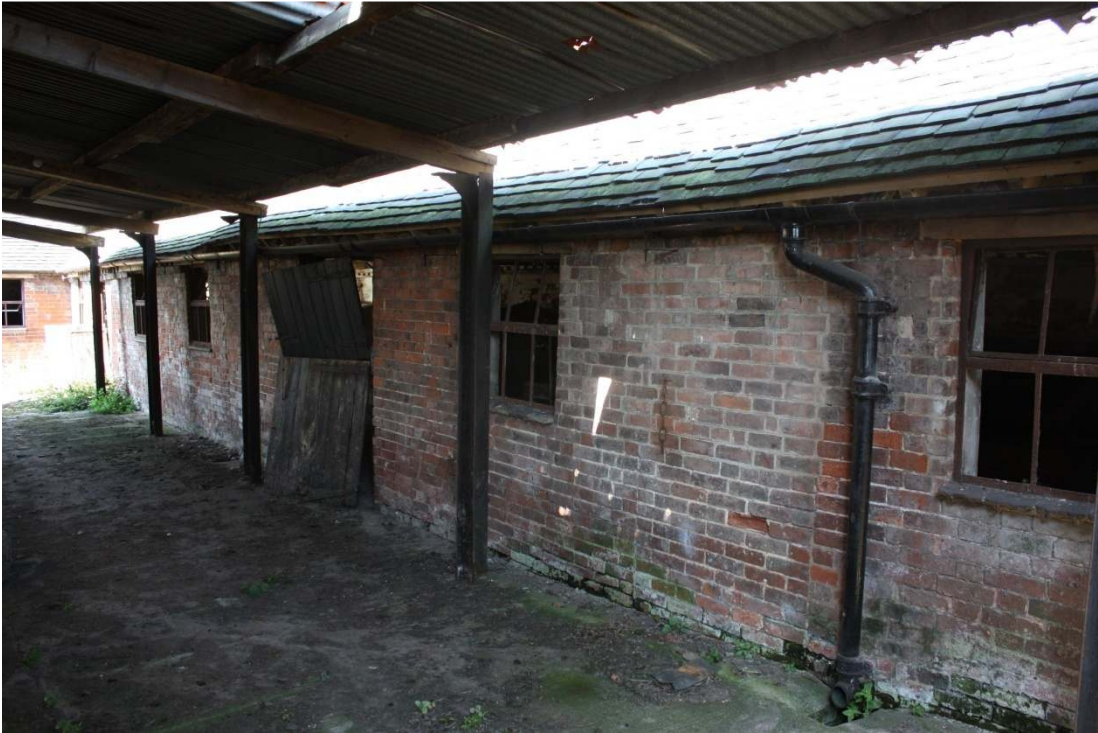
Plate 9: Exterior of the middle 7-bay section of cowshed range 2, viewed facing northwest
