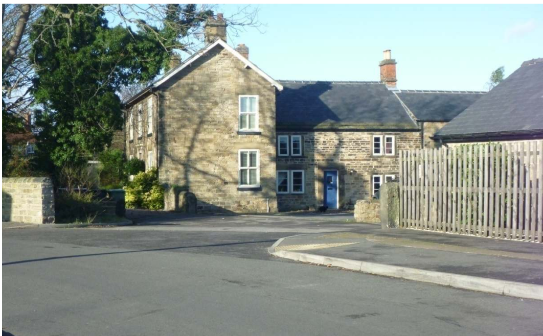
Plate 10: Grade II Listed Williamthorpe Hall Farm, viewed facing northwest
