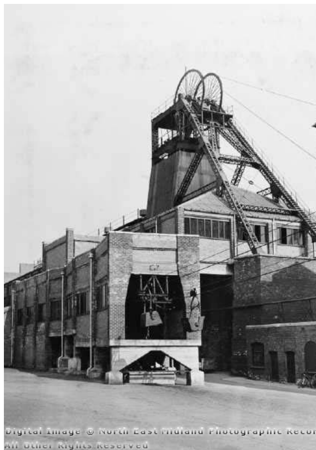
Plate 1: Photograph of the aerial ropeway station at the refurbished Williamthorpe Colliery, 1941
