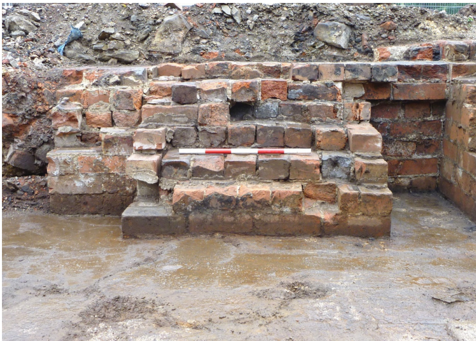
Plate 18 H1 (7003) looking south with Wall 7010 behind. 0.30 and 0.50m scales.
