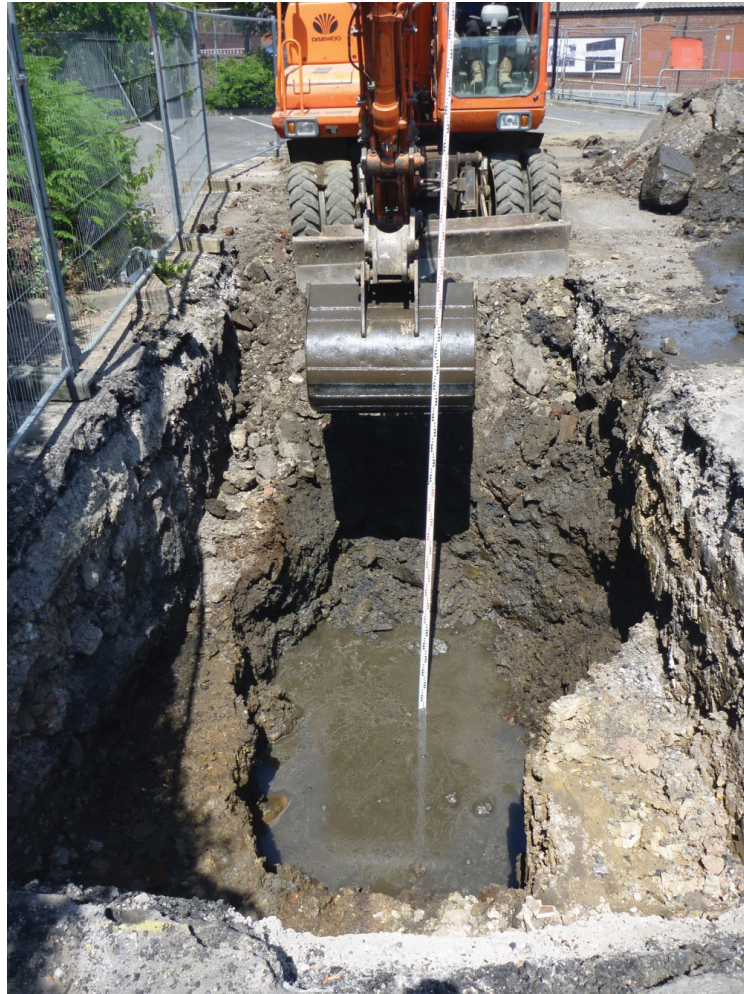
Plate 1 Working shot of machine excavation of palaeochannel (1011)
