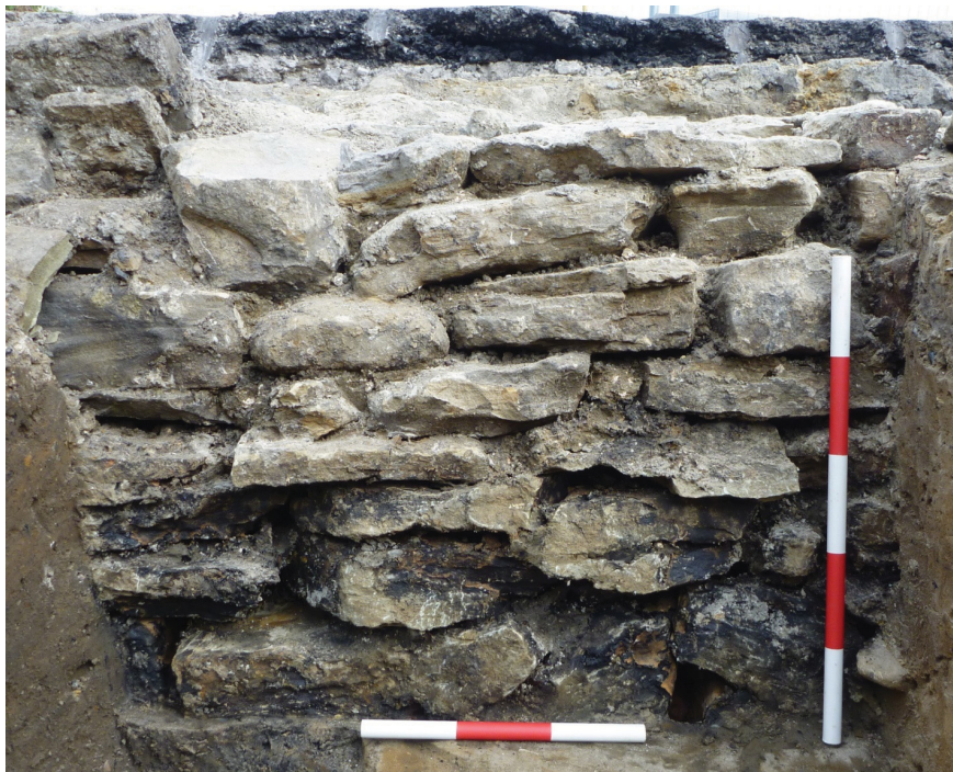
Plate 5 South face of wall 2012. 0.3 and 0.5m scales
