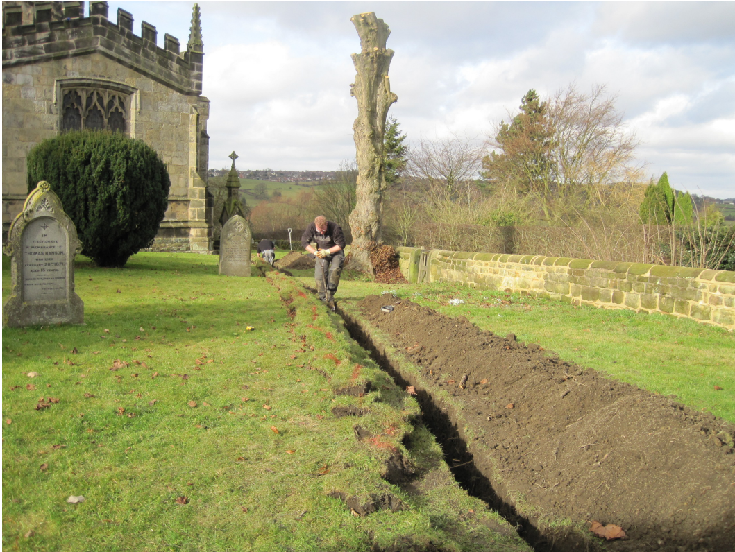
Plate 1: Excavation of service trench looking west
