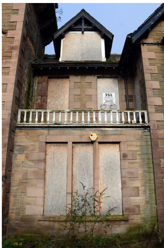
Plate 4: Later window replacing original loggia, south elevation (Shot 015)
