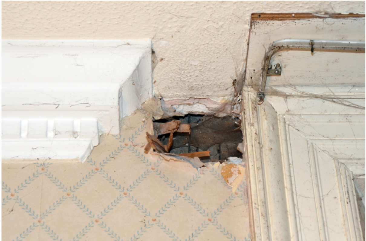
Plate 33: Late cornice in Room 20 and original window architrave (Shot 120)
