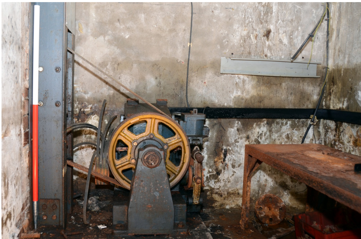
Plate 50: Lift gear in basement (Shot 201)
