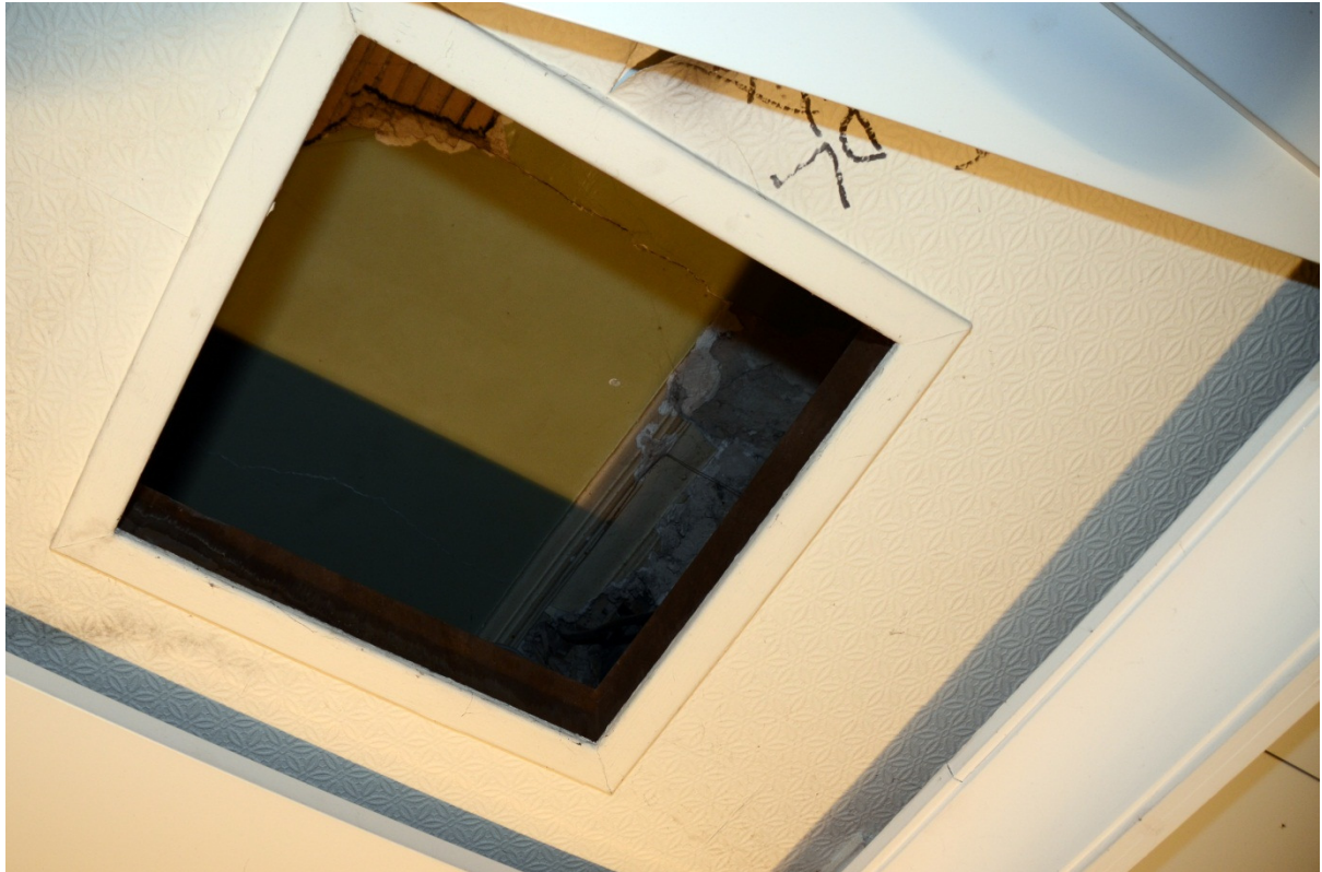
Plate 35: 1st floor hall hatch; original coving behind false ceilings (Shot 124)
