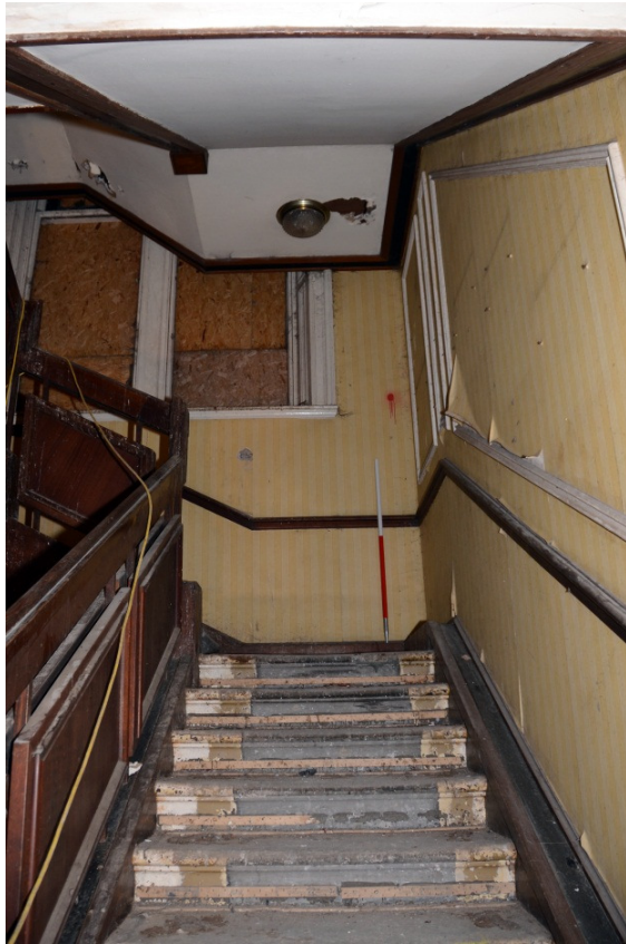
Plate 21: Stair from to 1st floor showing timber panels (Shot 134)
