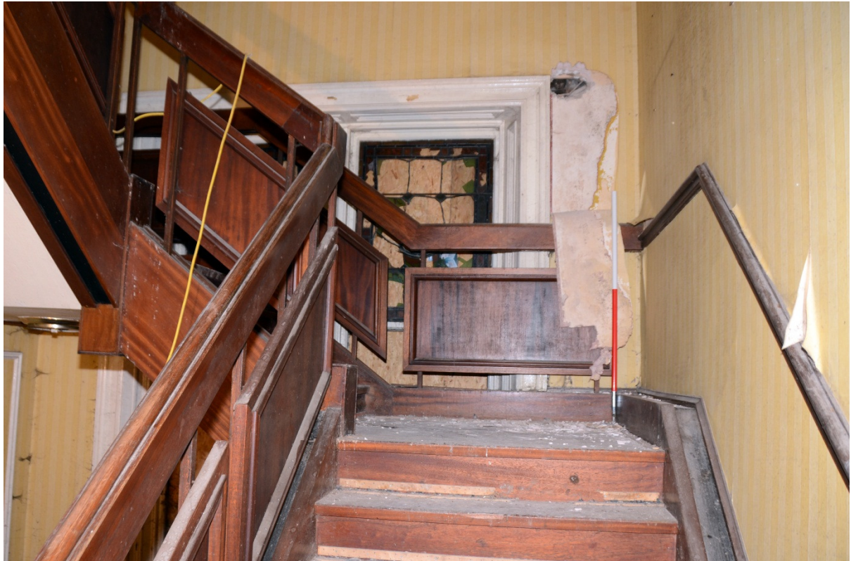
Plate 19: Stair to 2 nd floor obscuring original window (Shot 086)
