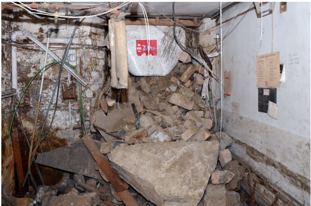
Plate 52: West wall of basement showing blocked chute (Shot 207)
