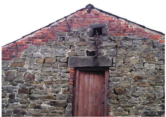
12. Detail of north eastern gable apex, showing owl hole and upper brickwork
