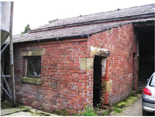
7. Detail of shippon extension brickwork, doorways and stone detailing
