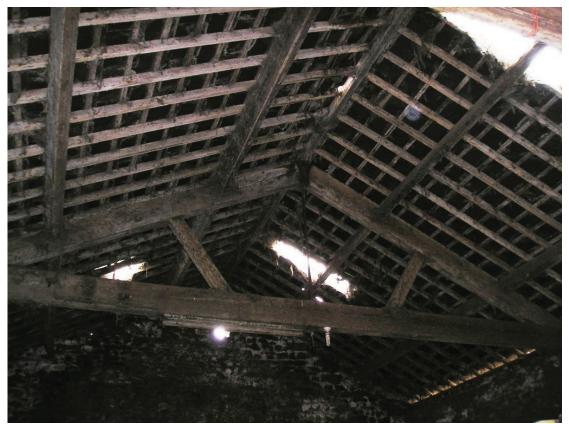
33. Roof truss with iron post and trenched purlins.
