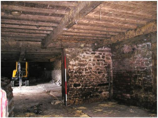
25. reverse view from within the extension bay looking into the main barn, showing doorway formed in former gable giving access between the two parts
