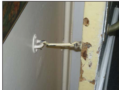
Figure 87: Hook and loop to hold doors open
