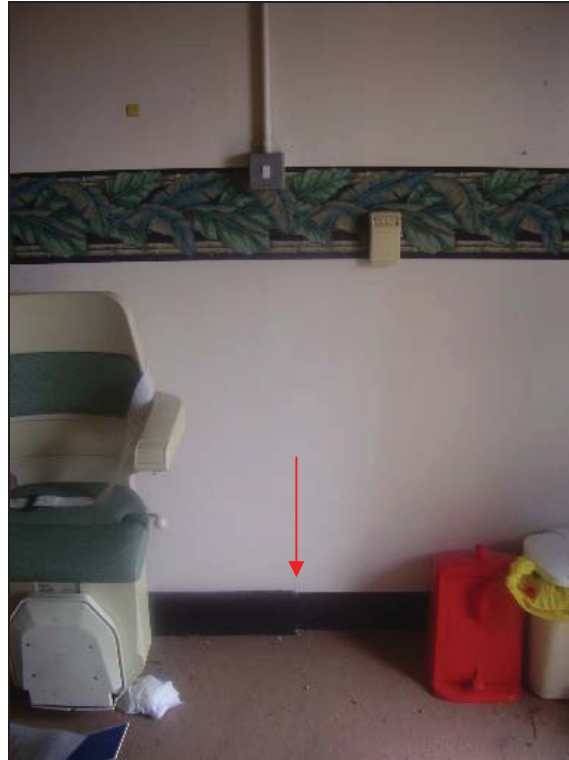
Figure 94: Chair lift and switch. Note the 'stepping in' of the skirting board just right of the chair.
