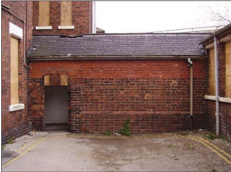
Figure 82: Phase 1 wall with phase 2 addition to wall and roof
