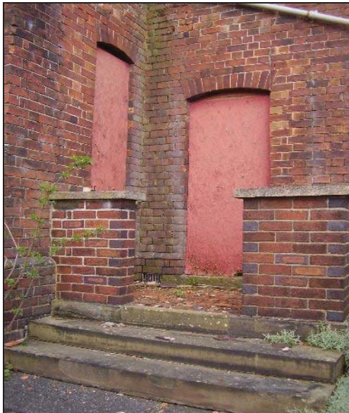
Figure 18: Possible scarring around west entrance, as shown by lighter brickwork suggesting outline of former lean-to porch (photo on right is key to photo on left).
