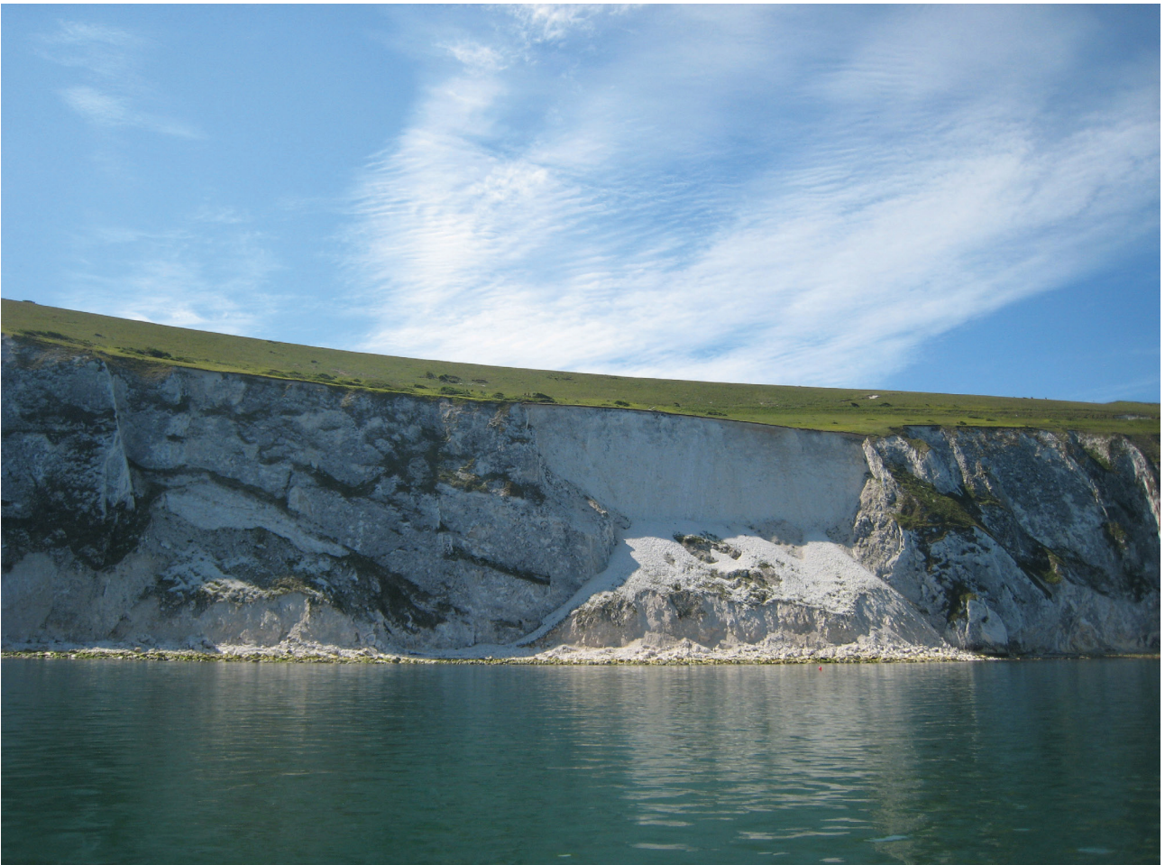
Figure 12. High chalk cliffs characterise the shoreline along the southern side of Alum Bay and are subject to on-going erosion resulting in significant landslips (Photo: Ine Demerre).
