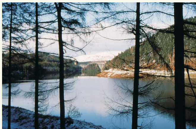
Fig. 4 The creation of reservoirs and the imprint of post-medieval and industrial period archaeology are a key association with some of the upland landform elements, such as at the Derwent Dams pictured here
