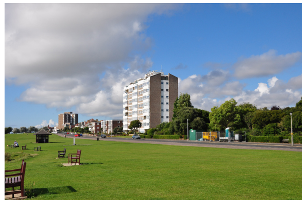
High rise buildings in Frinton
