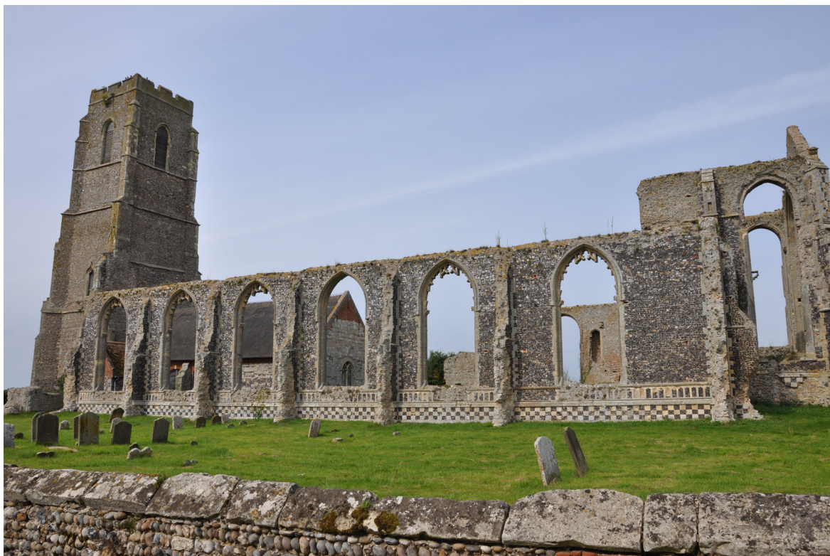
Covehithe church showing flint construction
