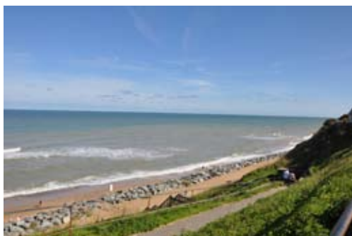
Rock berm at California
