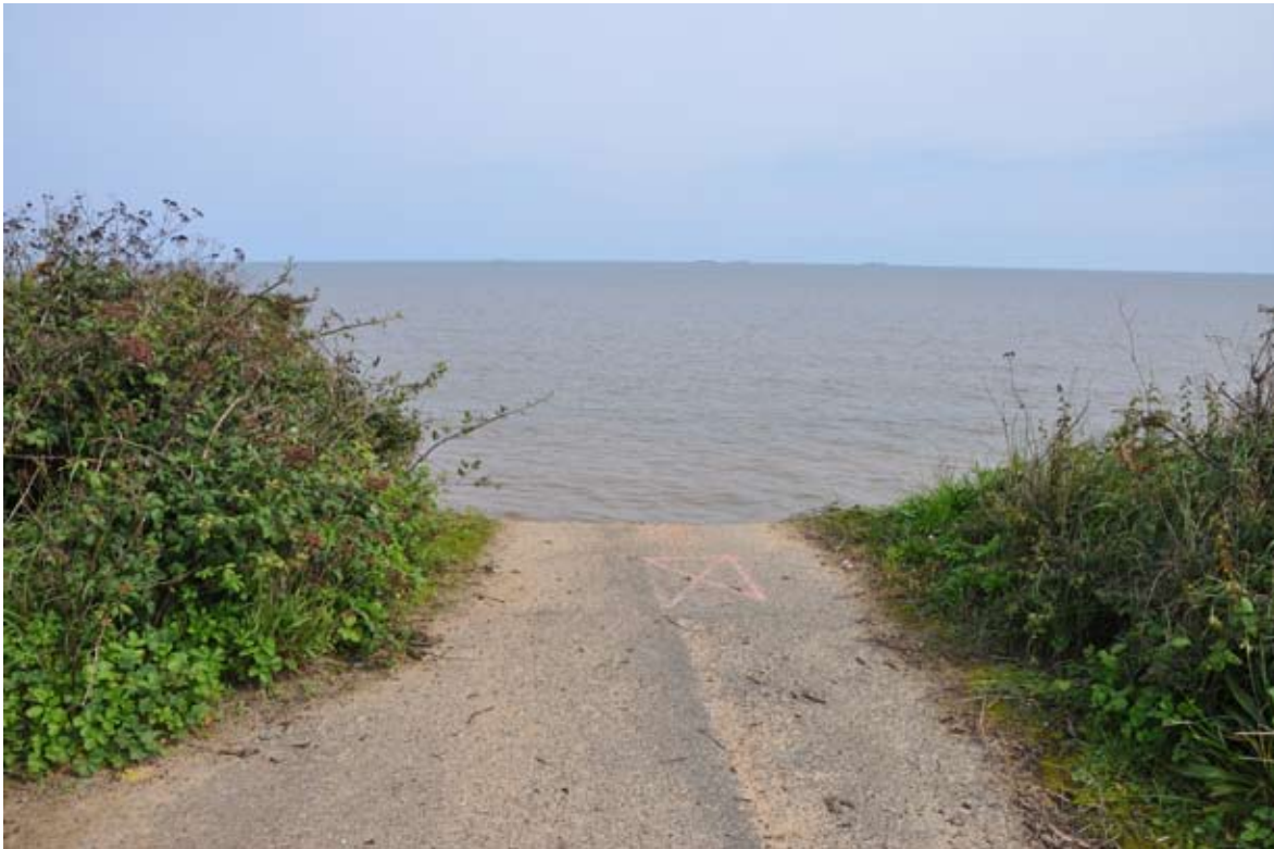
Road truncated by sea erosion near Covehithe
