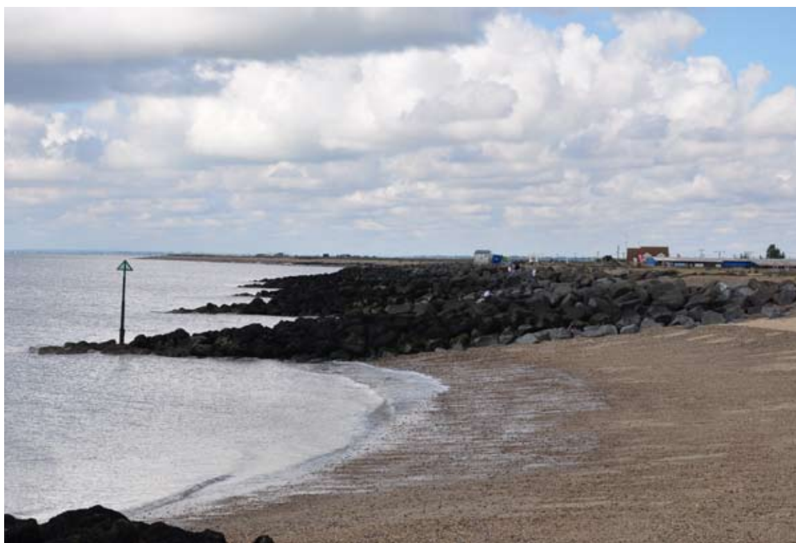
Breakwaters at Jaywick
