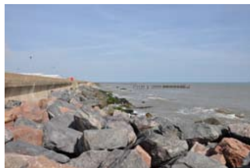
Seawall, rock armouring and old groyne at Lowestoft Ness
