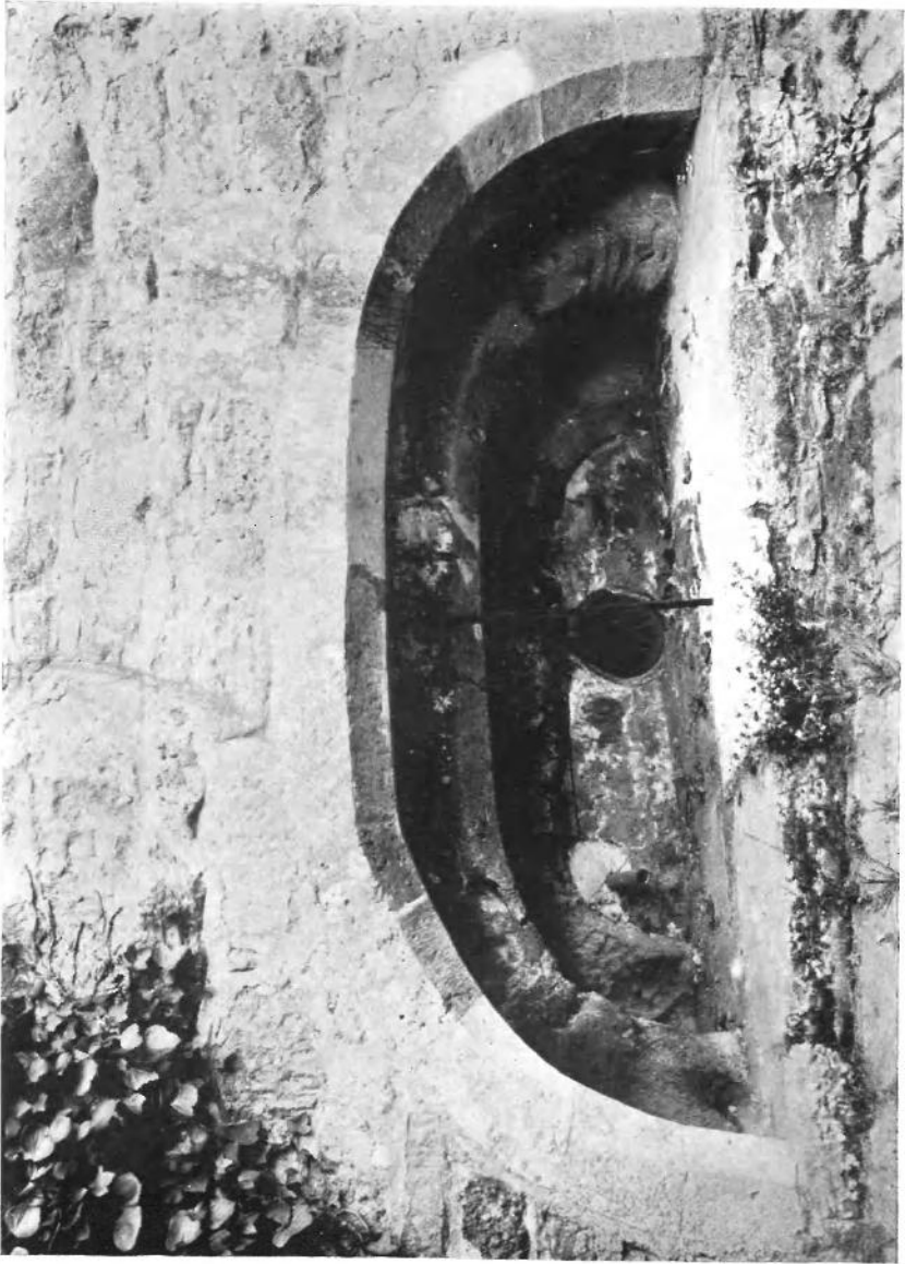
BEAULIEU ABBEY. SERVING HATCH BETWEEN THE KITCHEN AND THE PRAYER.
