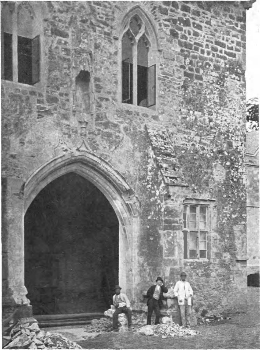
BEAULIEU ABBEY. SOUTH SIDE OF THE GREAT GATEHOUSE. Before "Restoration," from a photograph by the late Mr. W. J. C. Moens, F.S.A.
