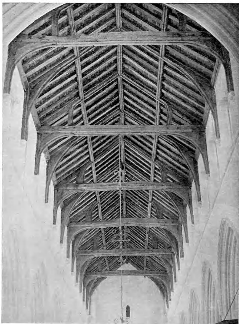
WALPOLE ST. PETER, NORFOLK : NAVE. COUPLE-CLOSE ROOF WITH RUDIMENTARY QUEEN-POSTS.
