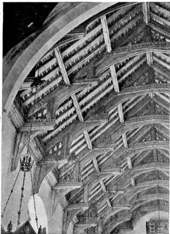
NO. I. WORLINGWORTH, SUFFOLK : NAVE. DOUBLE HAMMER-BEAM ROOF.
