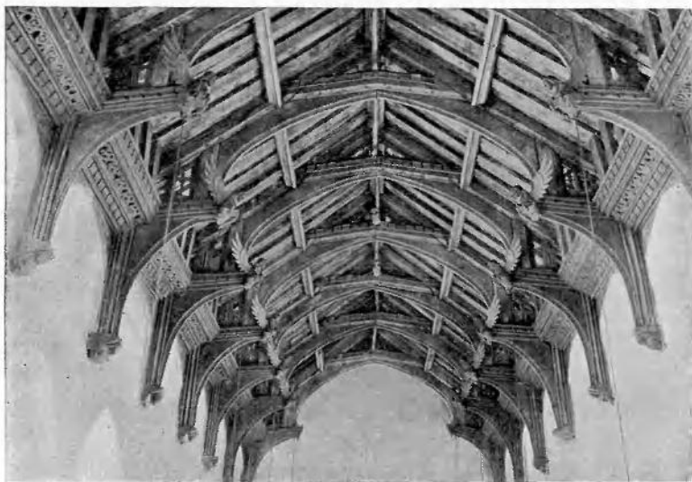
NO. 1. BADINGHAM, SUFFOLK : NAVE. HAMMER-BEAM ROOF, COLLAR TYPE.
