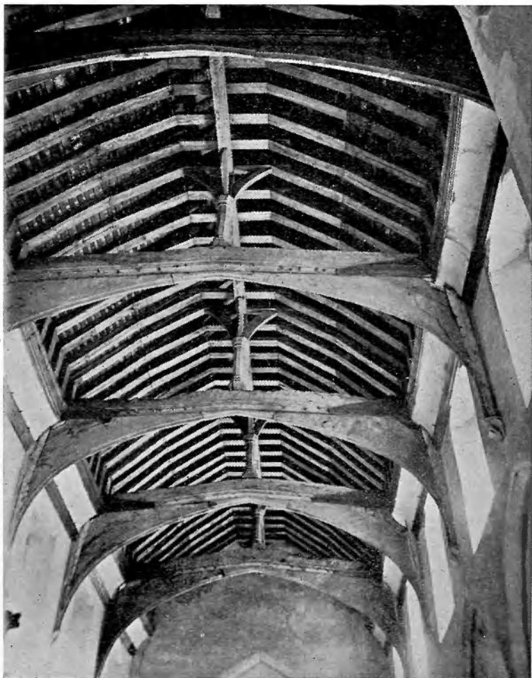
BARKING, SUFFOLK : NAVE. POST-AND-BEAM ROOF.
