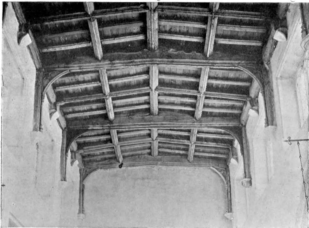
BLDINGTON, GLOUCESTERSHIRE : NAVE. FIRRED-BEAM ROOF.
