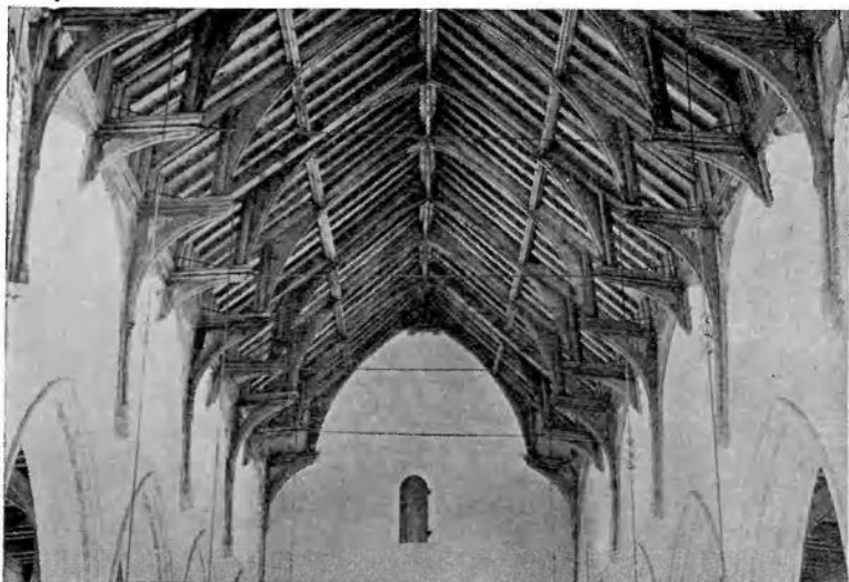
NO. 2. THORNHAM, NORFOLK : NAVE. HAMMER-BEAM ROOF, COUPLE TYPE.
