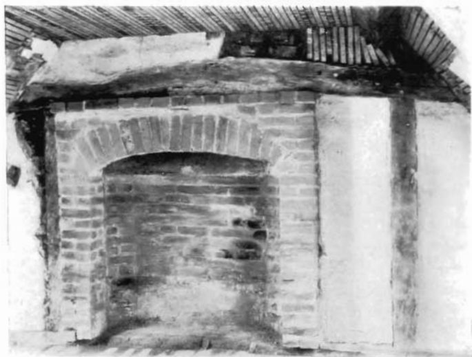
B. SIXTEENTH-CENTURY FIREPLACE (ARCH LARGELY REBUILT) IN ATTIC
