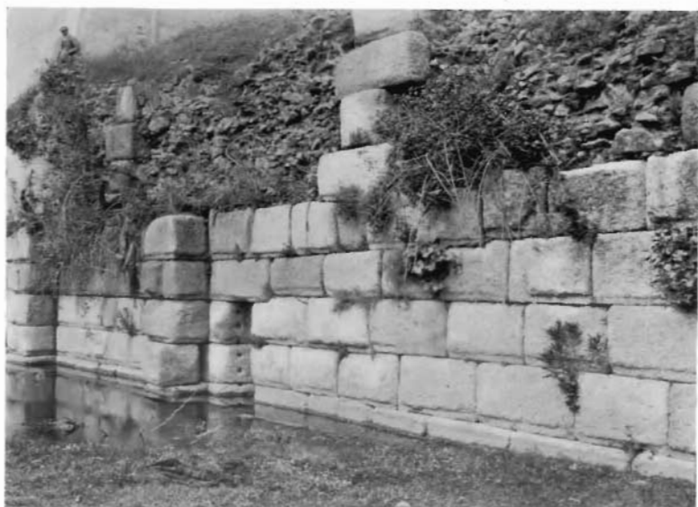
A. THE EMBANKMENT-WALL, MÉRIDA, BAYS 54, 55 Note the buttress-system and the sewer-mouth, with bar-holes.
