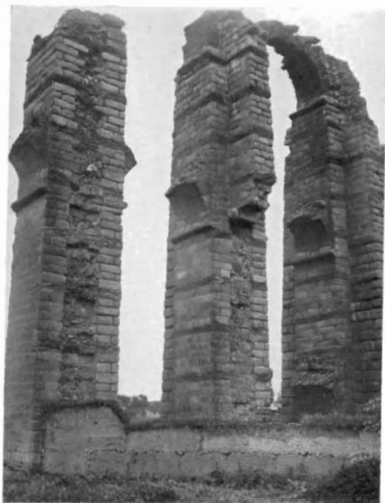
A. AQUEDUCT OF LOS MILAGROS, MÉRIDA Note relation of masonry to concrete and bonding-courses of tile
