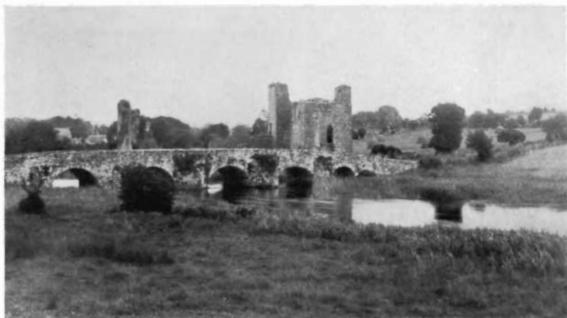
A. NEWTOWN TRIM : ST. PETER'S BRIDGE AND CROUCHED FRIARS
