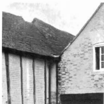
A. VIEW SHOWING JUNCTION OF ROOFS IN EAST WING
