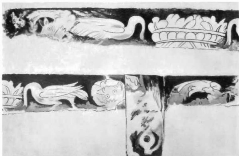
A. REMAINS OF WALL-PAINTING ON PARTITION-WALL OF WEST WING. 47, HIGH STREET, AMERSHAM
