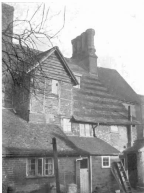
A. BACK VIEW OF NO. 61, HIGH STREET, AMERSHAM, SHOWING STAIRCASE TURRET
