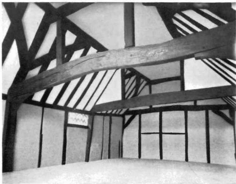
B. UPPER FLOOR OF WEST WING LOOKING N. 47, HIGH STREET, AMERSHAM
