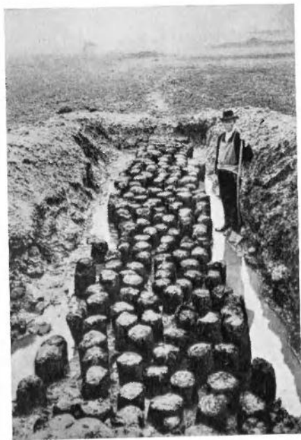
B. PILE FOUNDATION OF RAETIAN WALL IN MARSH NEAR DAMBACH ( O.R.L. , Str. xiii, Pl. xii, 5)
