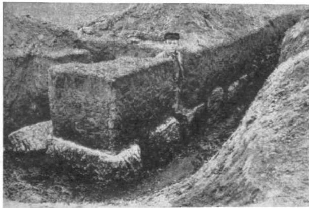
B. FOUNDATIONS OF THE WALL AT THE SULZACH, WITH GAPS TO LET FLOODWATER THROUGH ( O.R.L. , Str. xiii, Pl. xii, 4)
