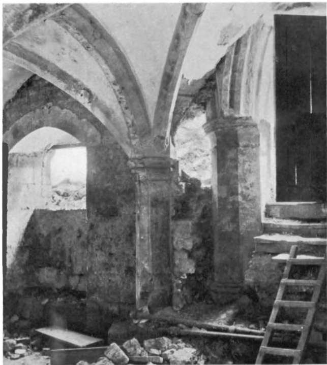
B. GREY FRIARS, LINCOLN. PIER OF ORIGINAL NORTH ARCADE AND RESPOND AND VAULTING OF LATER UNDERCROFT
