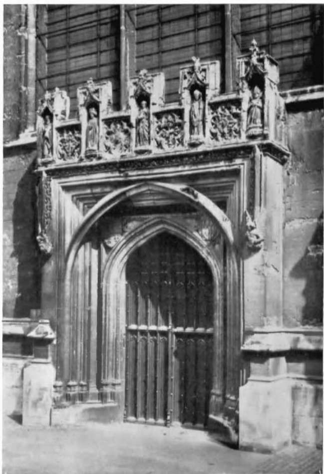
B. MAGDALEN COLLEGE, WEST DOORWAY OF CHAPEL (1474/8) DESIGNED BY WILLIAM ORCHARD
