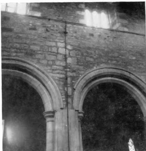
B. Early Saxon west wall in section in N. arcade
