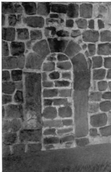
A. Jarrow, blocked N. door of chancel
