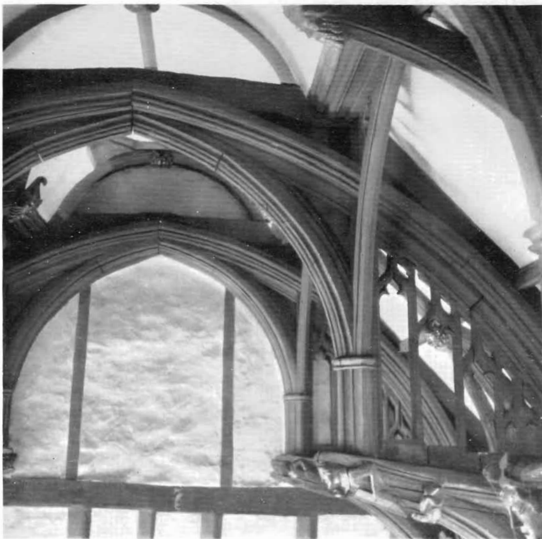
A. Roof truss
