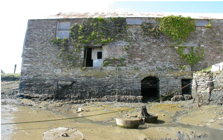
The East wall at low tide showing the sluice openings at Basement level.
