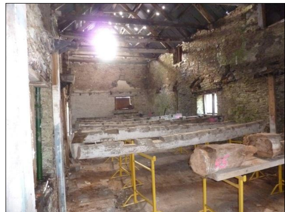
First floor beams cut down looking south with rotten stumps retrieved from the wall in the foreground
