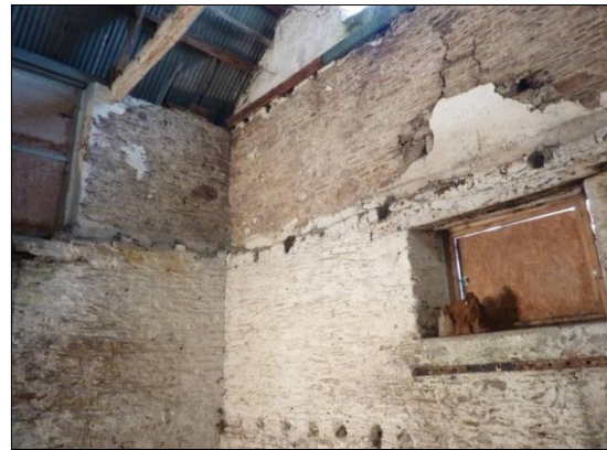
Joist holes in the lower part of the south wall for adaptation for office
