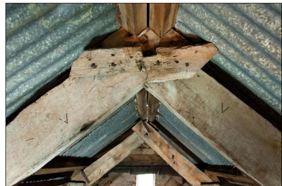
Looking south: apex truss V
