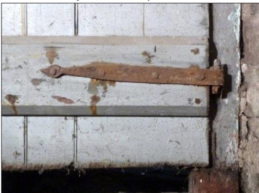
Detail of early hinge on the inside of ground floor door D2
