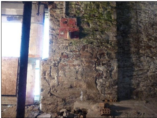
Early 20th century blocked Fireplace in the east wall
