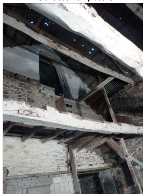
Looking from ground floor up north east through 2 first floor to door D5 and roof. First floor Beams 1 and 2 with roof tie beam D above
