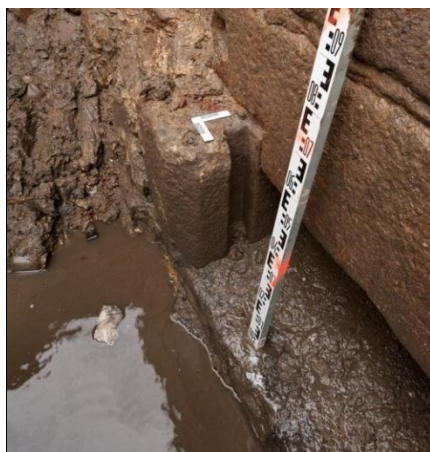
Details of Sluice S3: seating for sluice boards possibly 16th century
