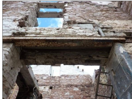
Detail of Doorways D4 above and D3 below showing steel lintel and re-used mill lintel. Looking north
