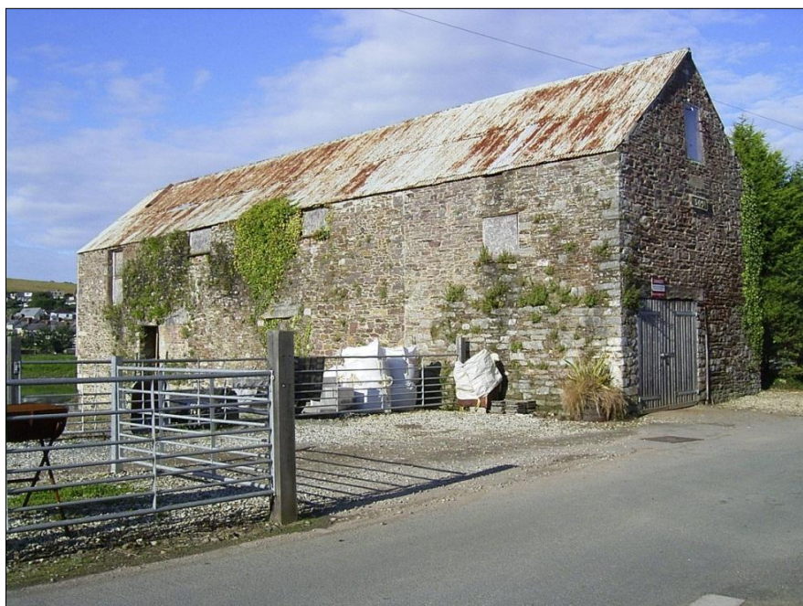
The mill from the north east showing the 19th century Extension with cart door onto the road and date stones for 1861 and 1598 in the wall above
