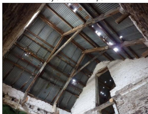
Extension looking into roof showing iron ties on trusses and the original north wall of main mill building
