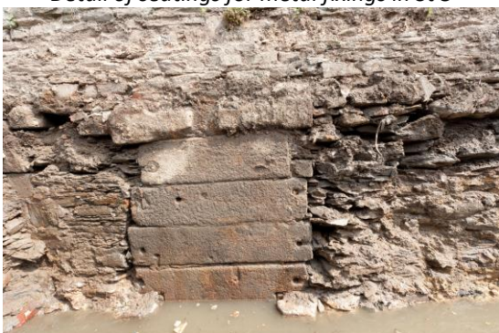
Re-used stones in outer blocking of S3 west sluice with 16th century sill as lintel
