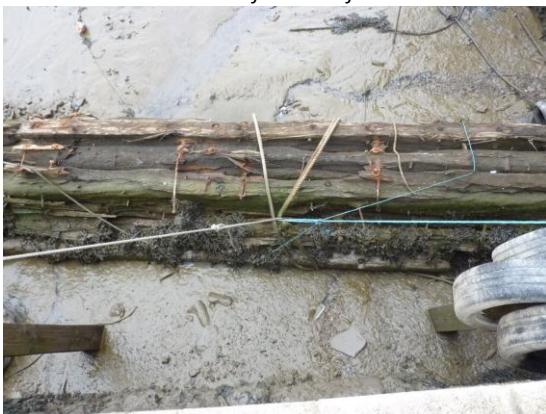
Pontoon showing iron bolts and spikes
