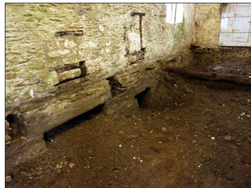
Looking northwest: S3 (left) and S4. Joists J3 and J4 removed, J5 beyond. Blocked sluice controls F2 & F3 in the wall above
