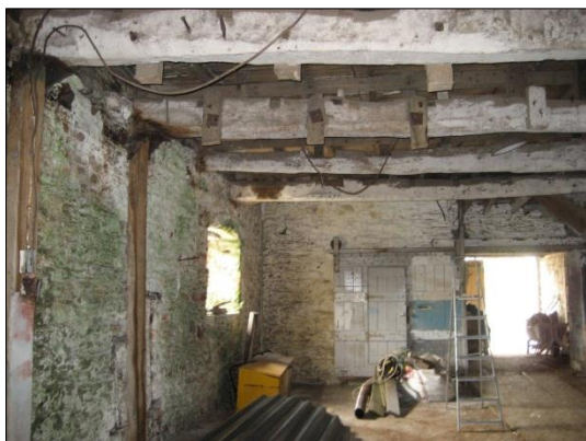
Ground floor looking north with Beam 4 in foreground. Remnants of a wooden hopper from the upper floor showing as sawn off vertical timbers
