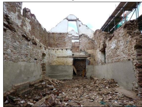
Looking north with roof and all internal timbers removed . Lower walls part plastered for tanking.
