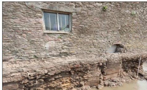
West face foundations and blocked sluices
