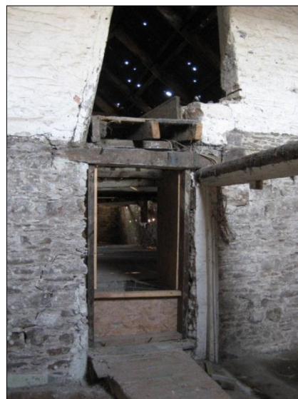
Detail of doorways D5 and D4 with partial remains of the sack ramps
