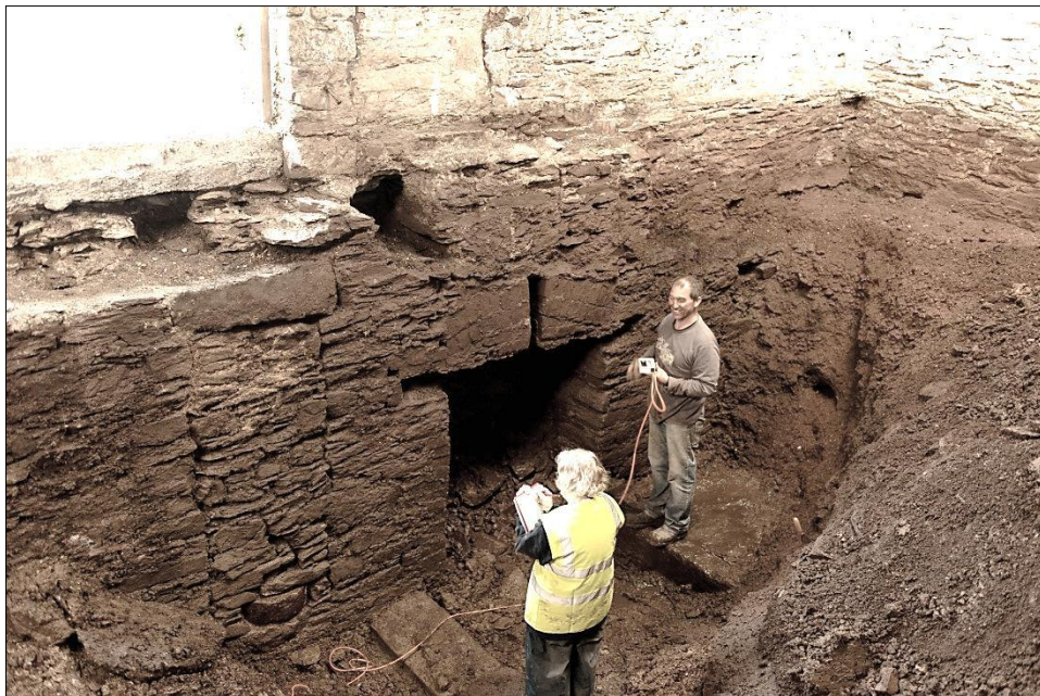
Basement Interior: east wall with blocked sluice S2, brick arch of sluice S5 and pitched paving on floor to right
