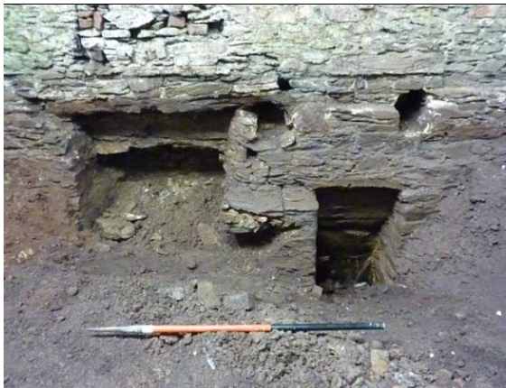
Sluice arch S5 and S2 West arch
