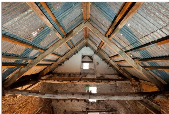
Roof structure looking north
