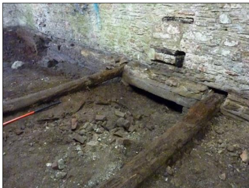
Looking south west: ground floor joists, J3 (with scale) and J4 on each side of sluice S3 lintel. Blocked sluice control F2 in the wall above
