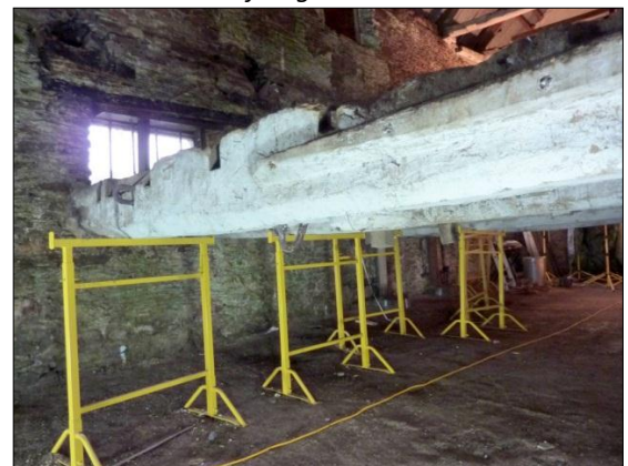
First floor beams cut down with Beam 5 in foreground. Note the iron hasps in the side and underneath which would have been used to lift the mill stones for dressing.
