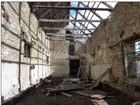
Looking north with roof being removed
