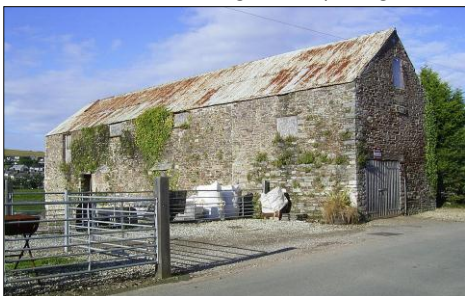
East and north faces showing Extension
