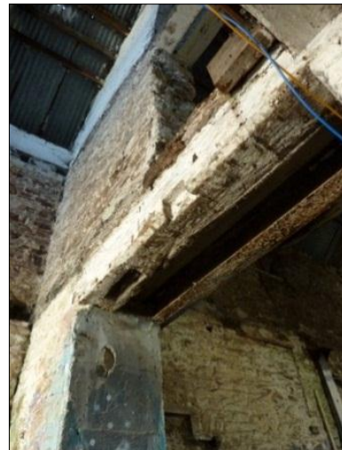
Looking up to wooden lintel and steel joist of door D3
