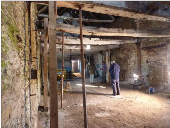
Ground floor looking north
