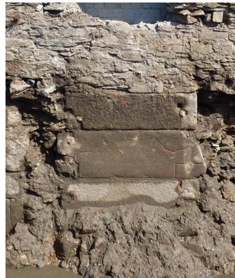
The granite blocking of 19th century sluice S5: this blocking is also made up of granite slabs which may have been capping stones
