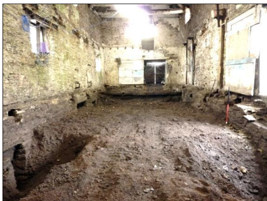
Looking north: ground floor joists removed. Showing the surface of the clinker fill in the Basement at the south end
