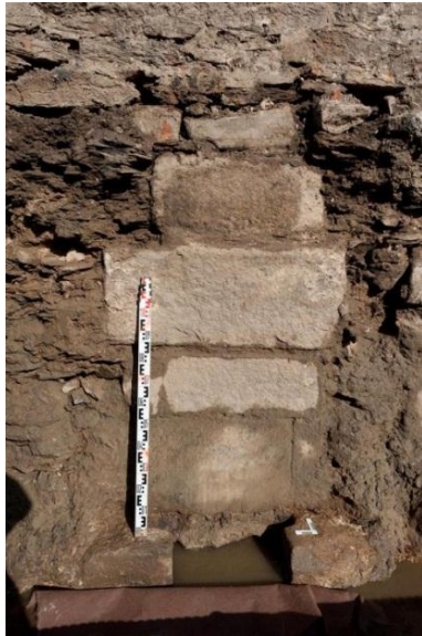
The granite blocking of Sluice S2. This small sluice which was probably part of the 16th century mill has rather less elaborate sluice board stones at the base but no lintel over the blocking
