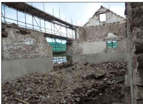
South east corner
