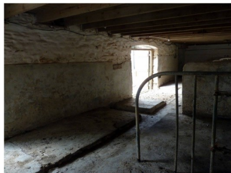
8 Egloserme A Cow House slurry channel and door DG4
