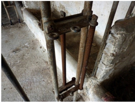
11 Egloserme A Cow House- adjustable tethering rods
