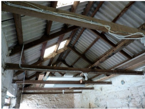
03 Egloserme B Cow shed- roof trusses
