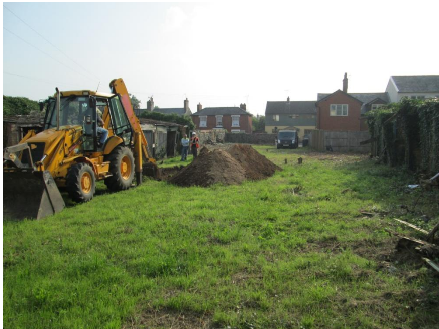
Plate 2. Pre-excavation, general site view, from the west
