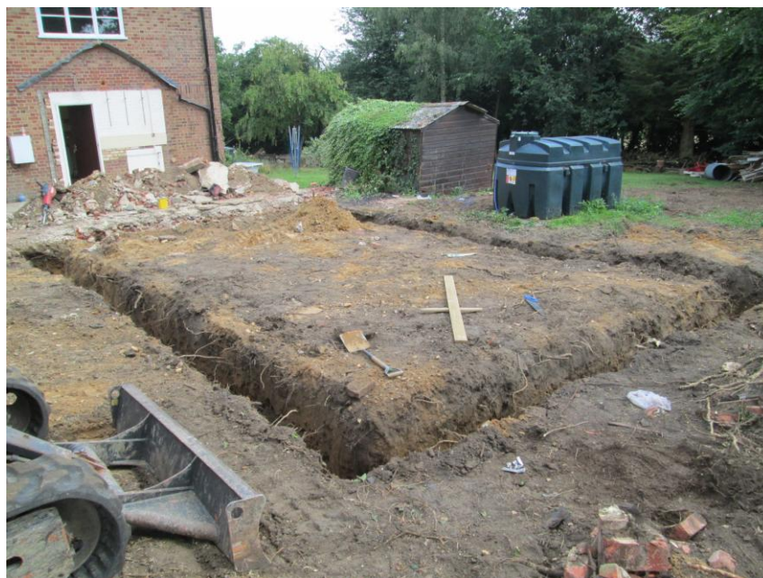
Plate 4. Post-excavation of garage footings
