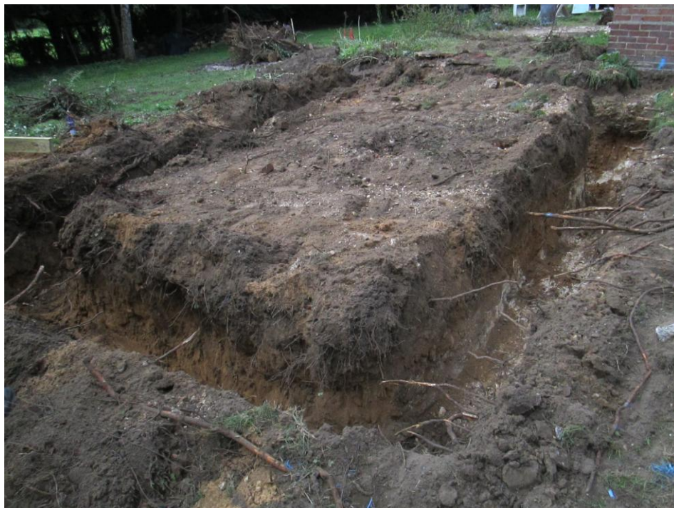
Plate 8. Post-excavation of part footings trench for extension (SS. 4)
