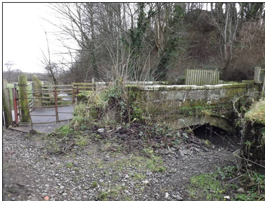
Plate 7: View looking east showing the small sandstone bridge over Scale Beck at the south end of the footpath to Workington Hall Mill
