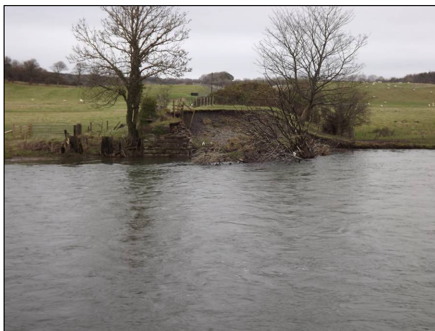
Plate 13: View looking east showing the remains of the bridge which carried the Cockermouth and Workington Railway across the River Derwent
