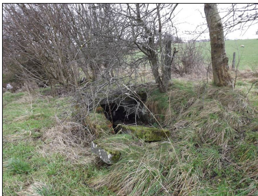
Plate 11: View looking south-east showing a brick and stone structure located along the north edge of the former Mineral Railway near Great Clifton
