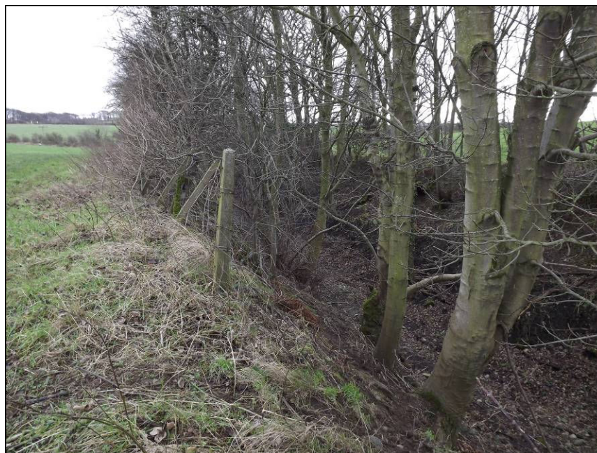
Plate 12: View looking south-east showing the surviving cutting for the former Mineral Railway line at the north-west end of the proposed pipeline route
