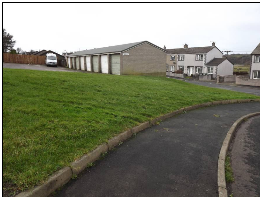
Plate 15: View looking east showing area of open land within the housing estate at Great Clifton where proposed groundworks will be undertaken
